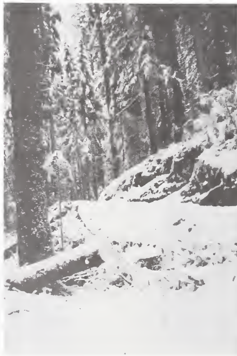
The road approaching Buck Springs Camp during that winter. The roads we constructed were not wide and allowed only a single vehicle to pass with turn outs quite close to each other for passing.
