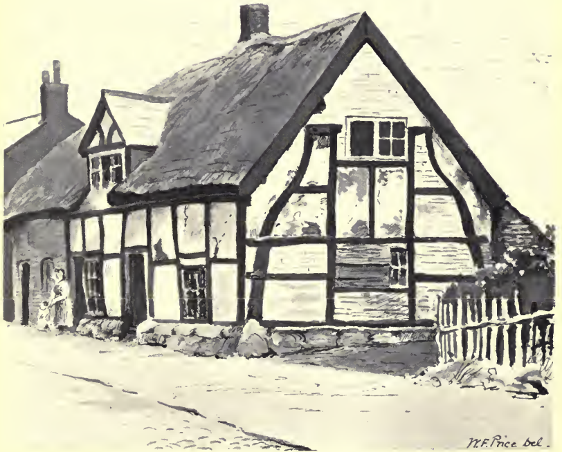
17TH CENTURY COTTAGE AT FARNWORTH, SHOWING TIMBER FRAMING. (Now taken down.)
