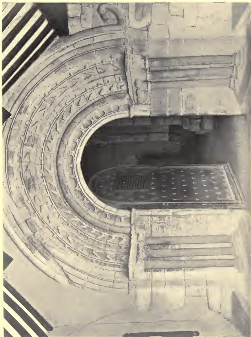
CARTMEL PRIORY CHURCH : DOOR OF NAVE.
