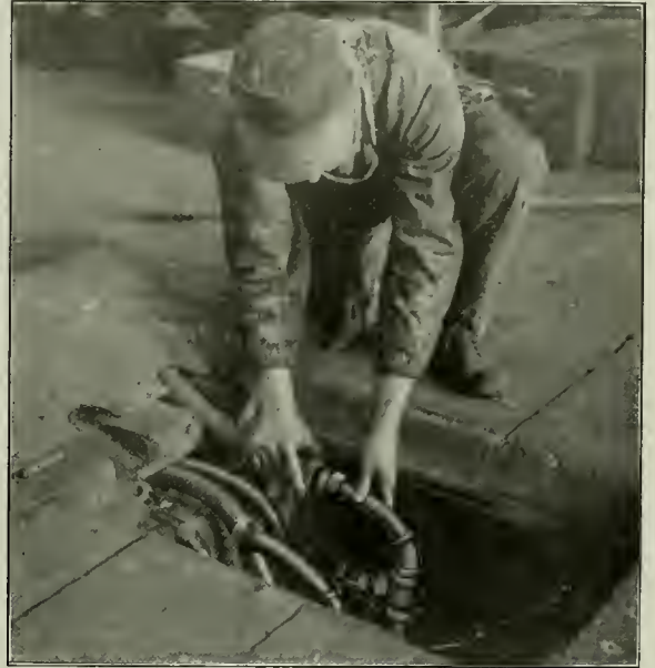
Fig. 8—Pipe Connections Placed at an Angle Away from the Operator When Making Connections
