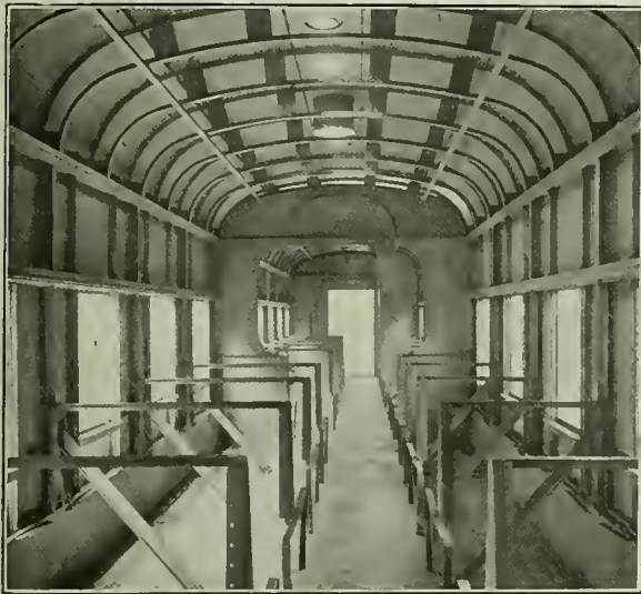
Interior of a Partially Finished Coach Showing the Steel Frame Work
