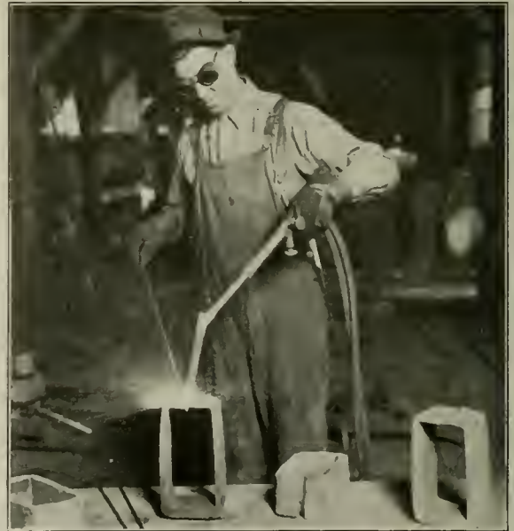
Welding Spring Bands At Rocky Mount
