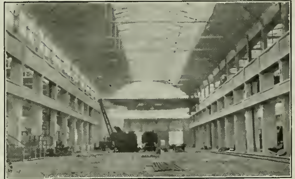
Locomotive Repair Shop at Nevers
