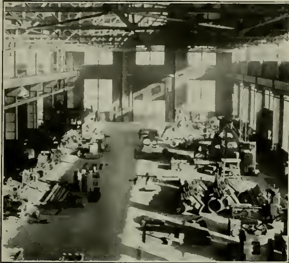
Frame and Cylinder Equipment in the South Bay
