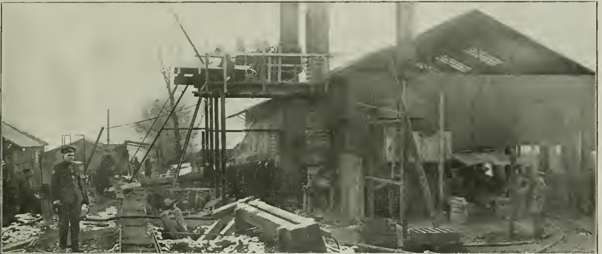
The Foundry as it Appeared in December, 1917; Note the Cupola Built Out of a Corrugated Furnace
