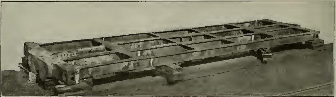
Repaired Cast Steel Tender Underframe
