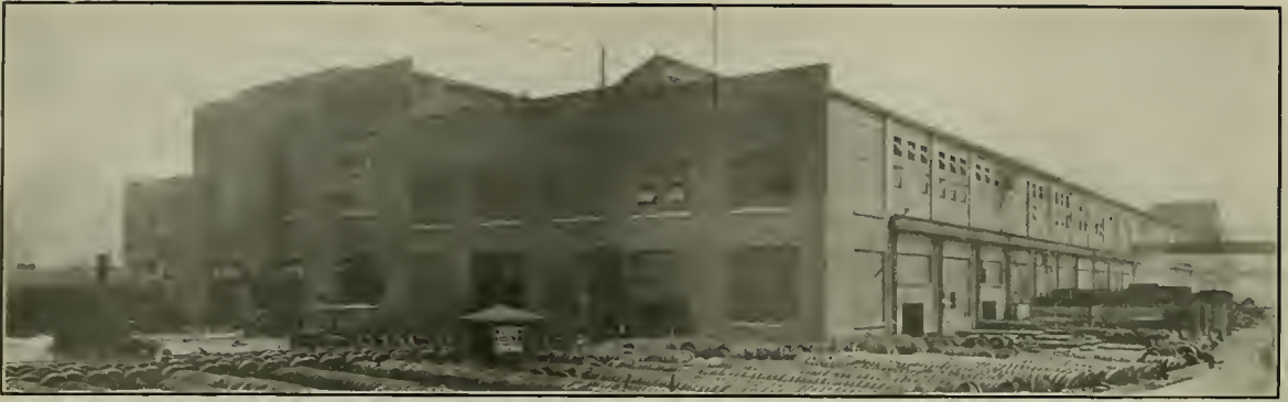
The Northwest Corner of the B. & O. Shops at Glenwood, Showing the Heavy Castings Platform at the Right
