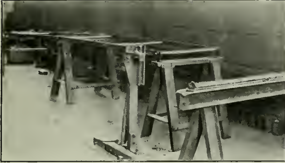
Fig. 6.—Roller Flue Racks Serving Second Hot Saw and Gaging Stand
