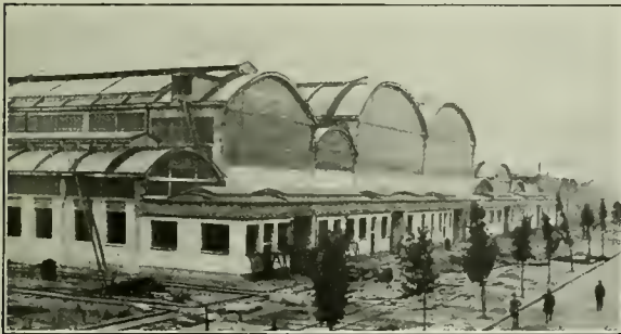
Locomotive Shops at Nevers
