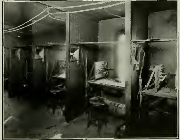
A Section of the School Equipment for Training Arc Welders
