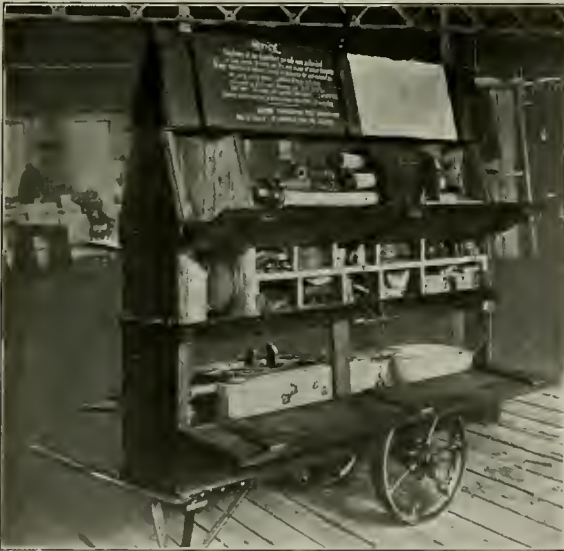
The Supply Truck Facilitates Making Quick Repairs
