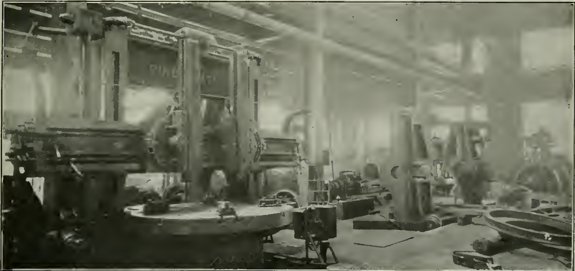
Part of the Wheel Shop Group
