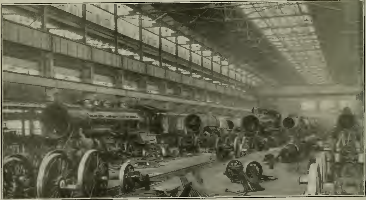
Interior of Erecting Shop
