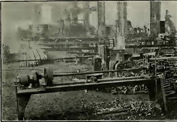
Looking South in the East Bay at the Flue Shop
