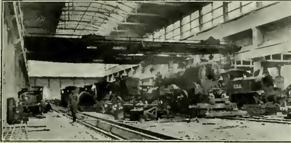
Repairing Locomotives at Nevers
