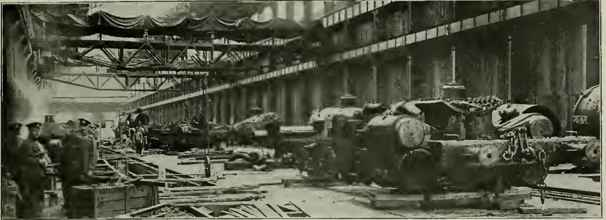
Machine Shop During Installation of Machine Tools, September, 1917
