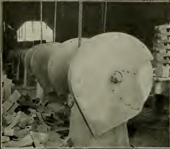
Fig. 3—Guards for Grinding Wheels
