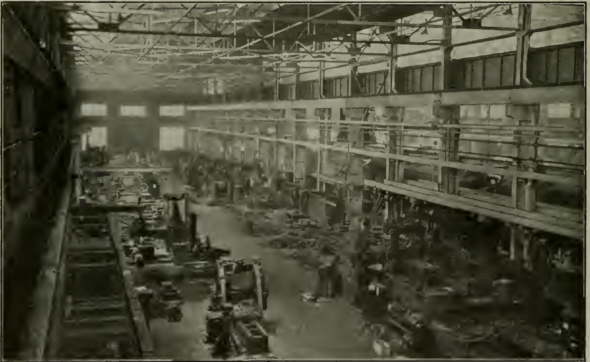
Looking North in the Heavy Machine Tool Bay Showing the Day Lighting and the Location of the Electric Lights
