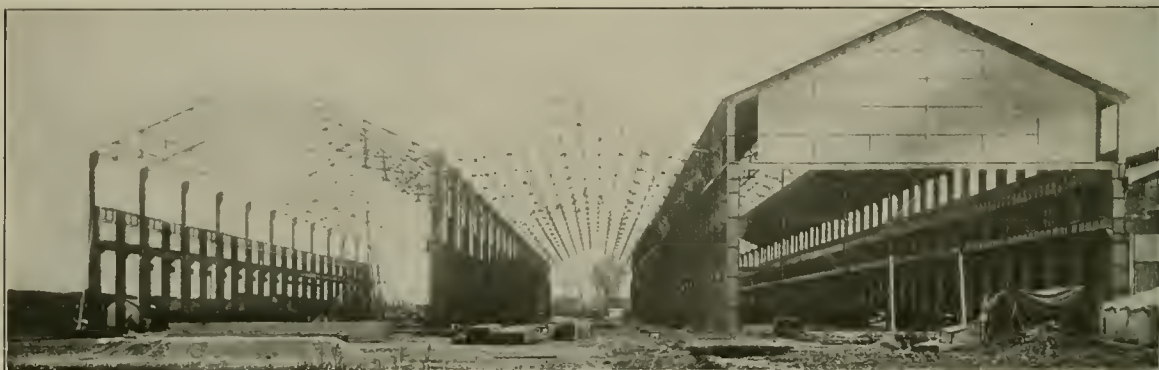
British Expeditionary Force Base Locomotive Repair Shops Near Rouen, France, As They Appeared in March, 1917; the Erection of the Outside Bay on the Left Was Started in February, 1917
