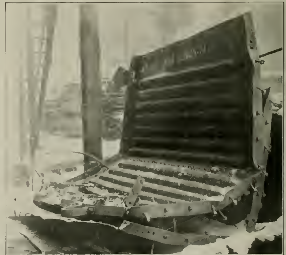
Steel Ends Removed from Destroyed Box Car
