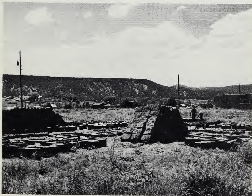
Making adobe brick, one of oldest New Mexico industries, is a waning occupation. However it is still being carried on by a few Indians, as shown here.
