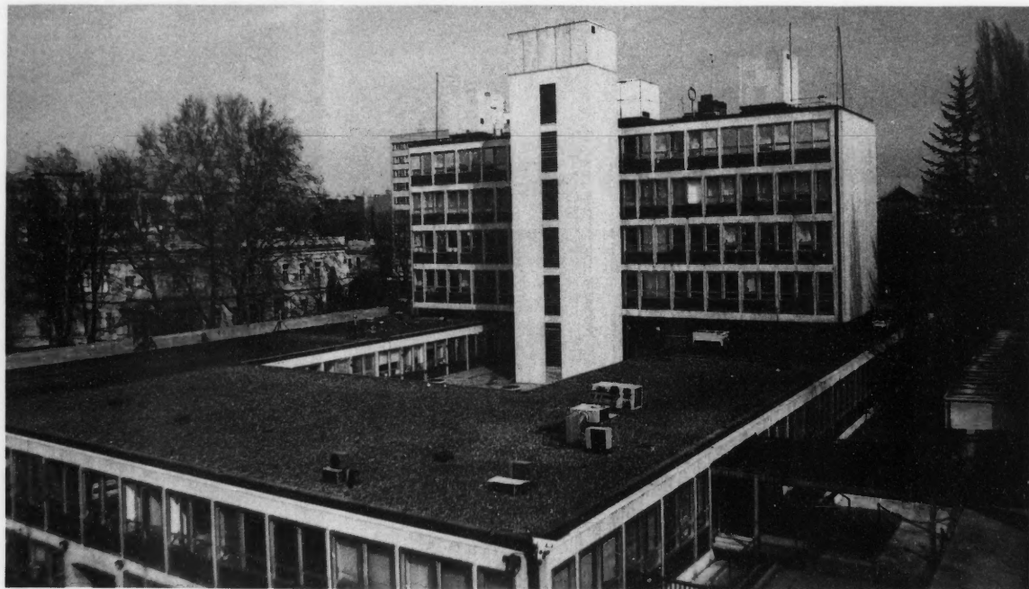
Rear of the embassy.
