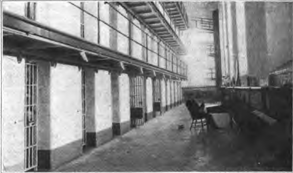
THE PREVAILING STYLE OF CELL-HOUSE—CELLS INSIDE The corridor is wide and airy, but the cells where the prisoners live out their lives are dark and unventilated steel cages, hot in summer and cold in winter
