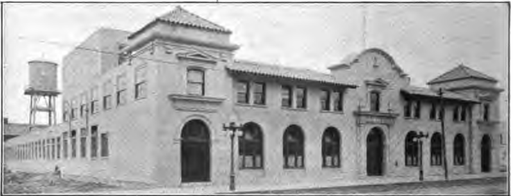
Sunaet Publishing Co., San Francisco, Cal., attractive Concrete building constructed with Hy-Rib, without forms.
