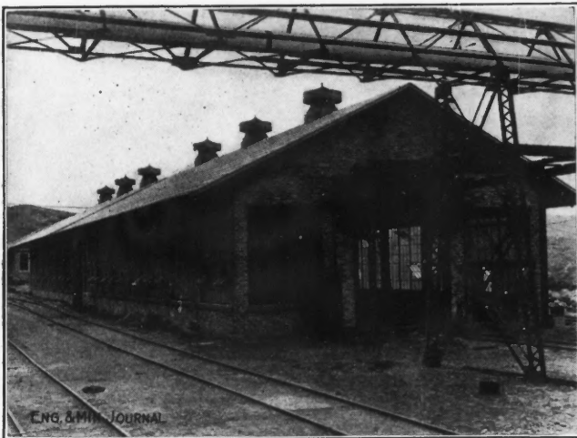
MECHANICAL SHOPS AT ARIZONA COPPER CO.'S NEW WORKS
