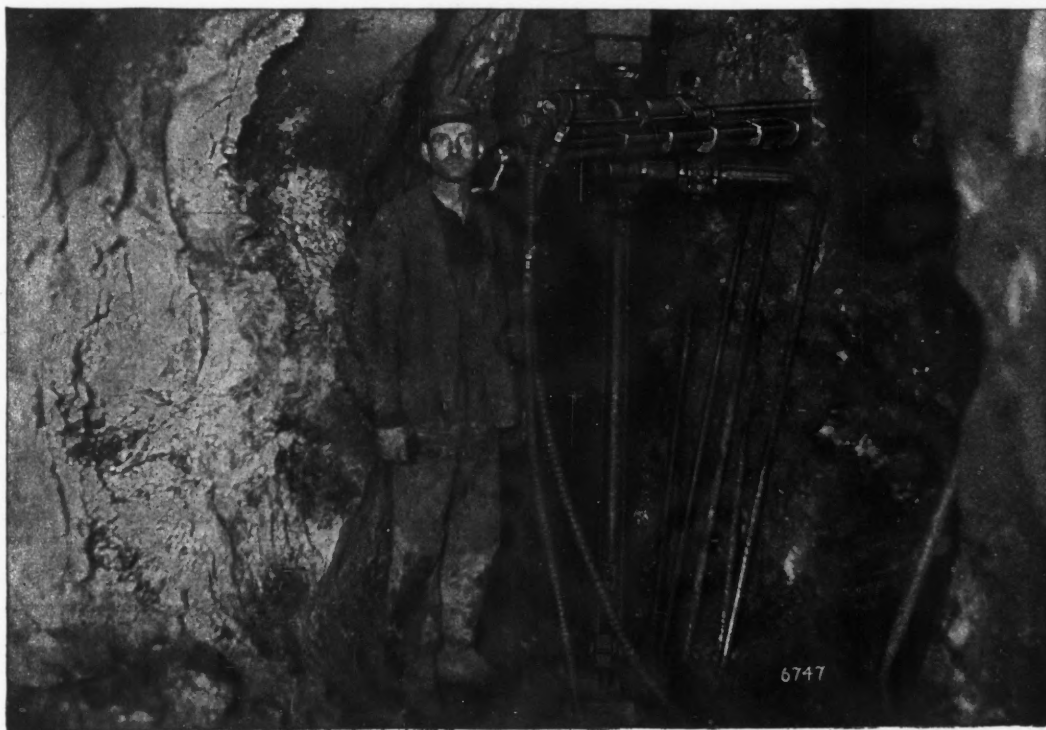
Leyner-Ingersoll Drill at Work on the 1500-Foot Level of the Golden Cycle Mine, Cripple Creek, Colorado.
