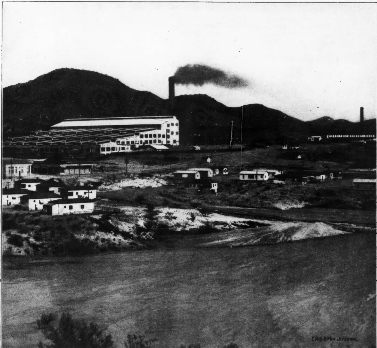
RAY CONSOLIDATED COPPER CO., 8000-TON MILL AT HAYDEN, ARIZ. The Hayden smelting works, to which the concentrates are sent, are situated back of the concentrator at the base of the big stack, the smaller stack directly in front of it being the power-plant stack.
