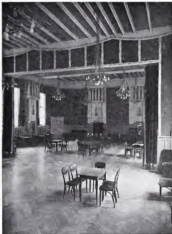
SMALL HALL, HAKESCHE HOUSE, BERLIN AUG. ENDELL, ARCHITECT
