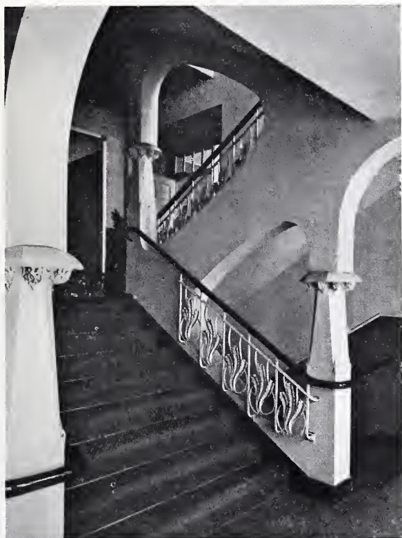
STAIRCASE OF THE HAKESCHE HOUSE, BERLIN AUG. ENDELL, ARCHITECT
