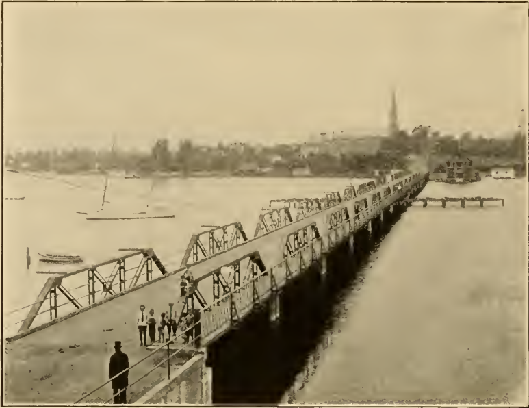
SPA CREEK BRIDGE, ANNAPOLIS, MD. (1100 FEET LONG)
