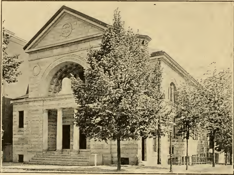
HEATING INSTALLATION IN THIS TEMPLE BY ENTERPRISE STEAM & HOT WATER HEATING CO.
