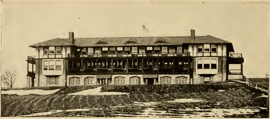
"EPSTEIN MEMORIAL" HOSPITAL HEATING, VENTILATION, ELECTRICAL AND WATER-WORK SYSTEMS DESIGNED BY PENNIMAN & FAIRLEY
