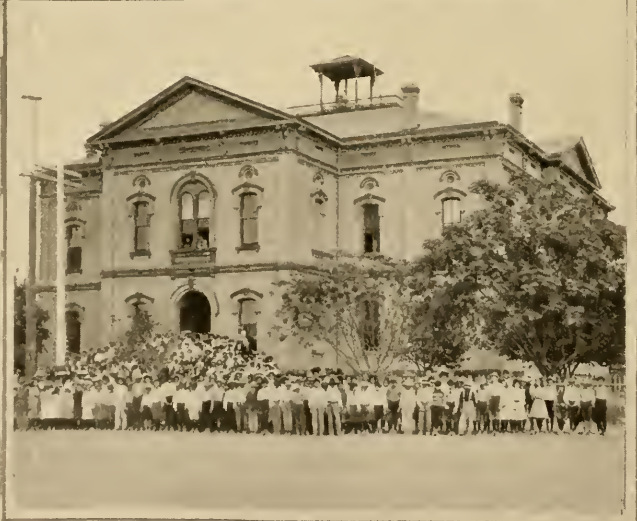
PUBLIC SCHOOL BUILDINGS OF TUCSON
