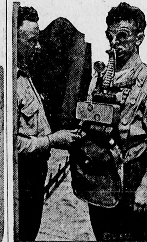
In order that the Chicago fire department may retain its efficiency, the local fire officials have been conducting a school to instruct the members of the department in the use of all the equipment with which a modern fire department is fitted. The photograph shows Chief Carnody showing a fireman how to use a rescue apparatus.
