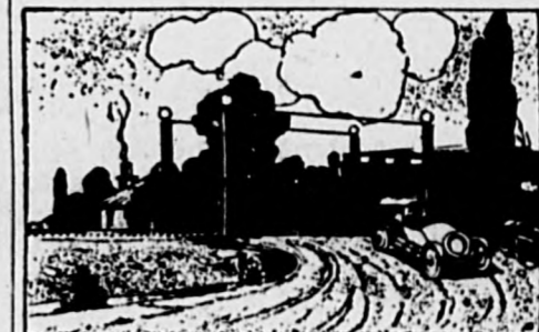
Spring Gates for Railroad Crossings, Which Drop Across the Road While the Lamps on the Posts Light Up.
