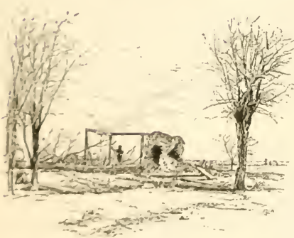
RUINS OF THE HENRY HOUSE. FROM A PHOTOGRAPH PROBABLY TAKEN IN MARCH, 1862.
