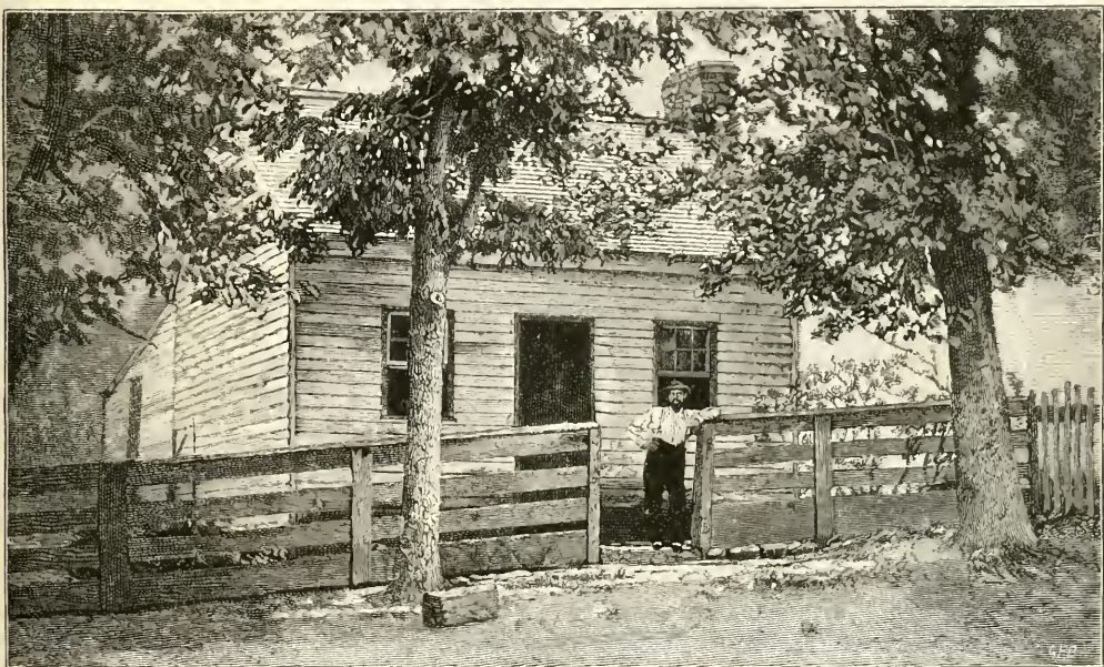
GRANT'S BIRTHPLACE AT POINT PLEASANT, OHIO. (1885.) THE HOUSE LOOKS UPON THE OHIO RIVER.
