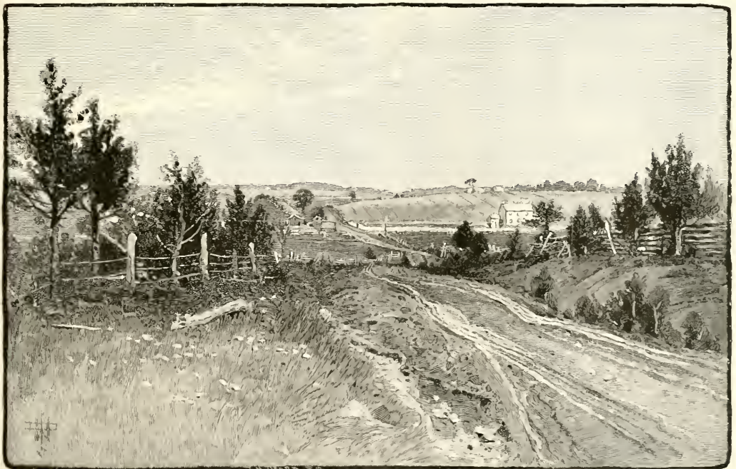
THE SUDLEY SPRINGS ROAD, LOOKING NORTH FROM THE SLOPE OF THE HENRY HOUSE HILL.
