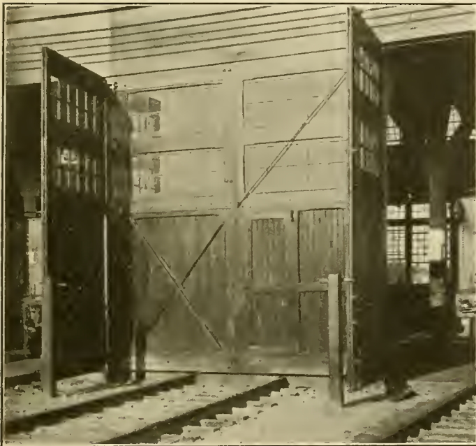
ENGINE HOUSE DOORS AT WEST SPRINGFIELD.
