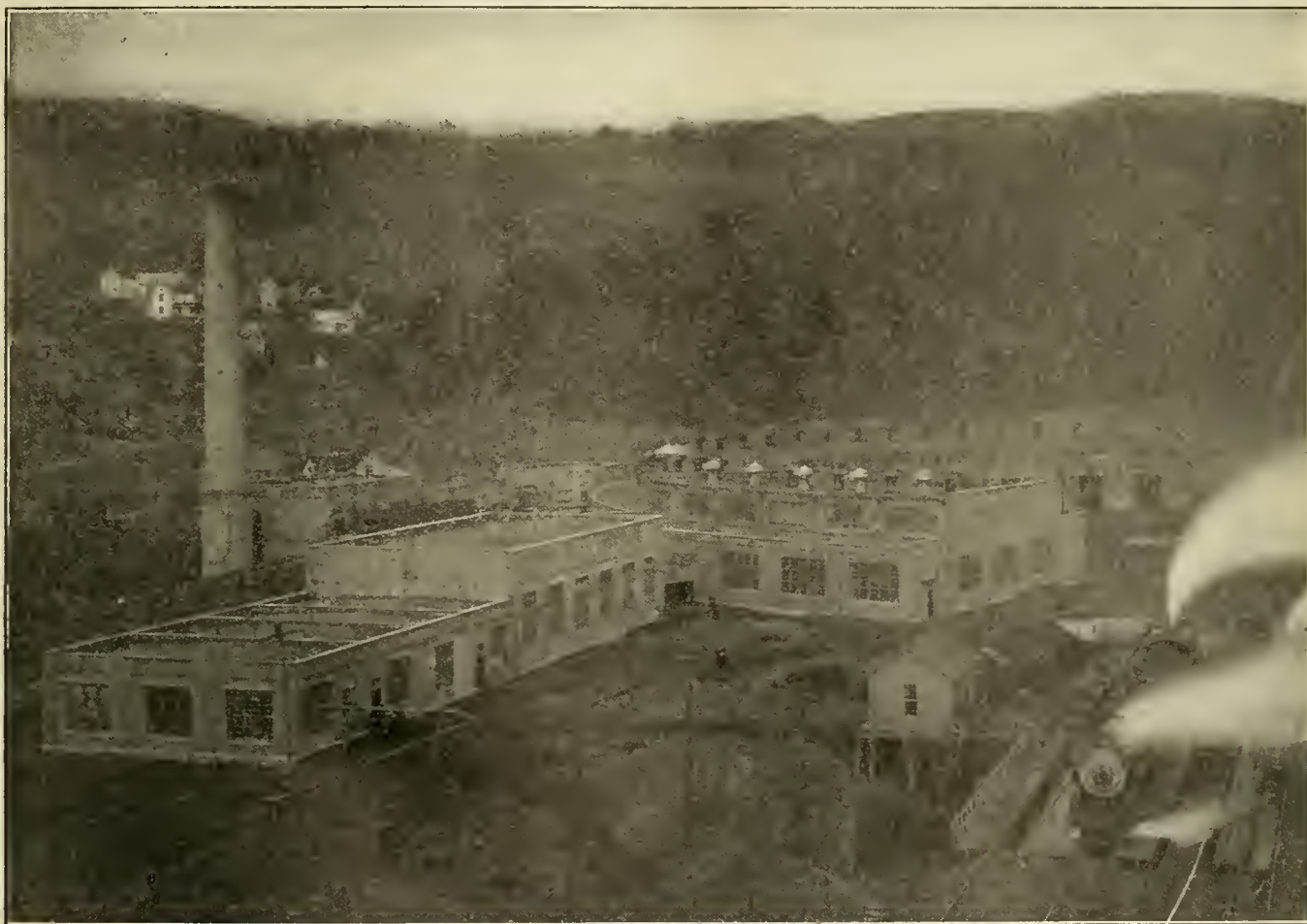
GENERAL VIEW OF THE NEW LOCOMOTIVE TERMINAL ON THE NEW YORK CENTRAL LINES AT CORNING, N. Y., TAKEN FROM THE TOP OF THE COALING STATION
