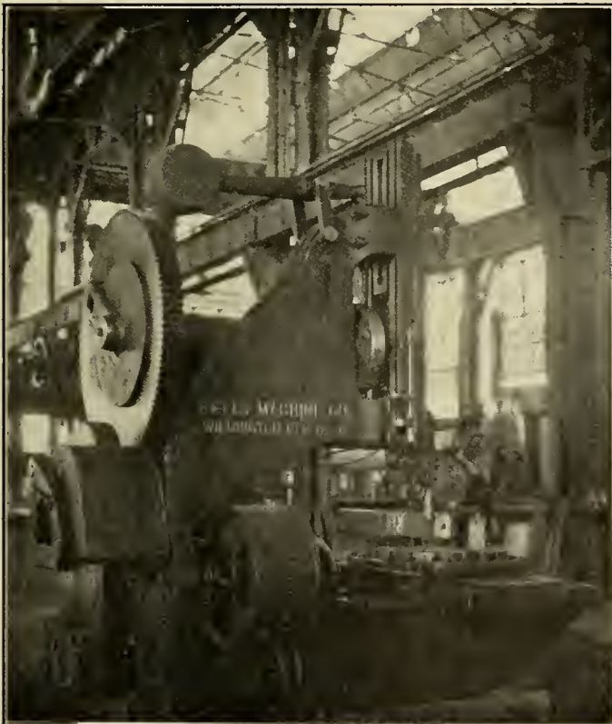
HEAVY SLOTTER WITH DIRECT ELECTRIC MOTOR DRIVE IN THE EMPALME SHOPS
