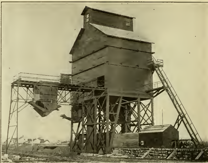
COALING STATION ERECTED BY THE ROBERTS & SCHAEFER CO. AT BARING, MO. THIS PLANT IS OF THE CHAIN AND BUCKET TYPE AND HAS A CAPACITY OF 500 TONS. THERE ARE TWO SUSPENDED WEIGHING POCKETS ON THE STATION PROPER, AND IN ADDITION THERE IS A STEEL BRIDGE WITH A 10-TON WEIGHING HOPPER FOR SERVING THE TWO MAIN LINE TRACKS. THIS HOPPER IS SERVED BY MEANS OF A 3-TON CAR, WHICH RECEIVES ITS LOAD FROM THE MAIN STORAGE POCKET. THE PLANT IS OF WOODEN CONSTRUCTION WITH THE EXCEPTION OF THE BRIDGE.
