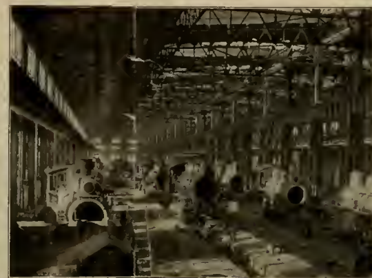
VIEW TAKEN FROM POINT B SHOWING THE GENERAL FITTING SHOP. IT WILL BE NOTICED THAT THE LOCOMOTIVES ARE SET STAGGERING, SO AS TO PERMIT THE EASY REMOVAL OF THE FLUES. THIS VIEW GIVES AN EXCELLENT IMPRESSION OF THE GENERAL APPEARANCE OF THE SHOP.
