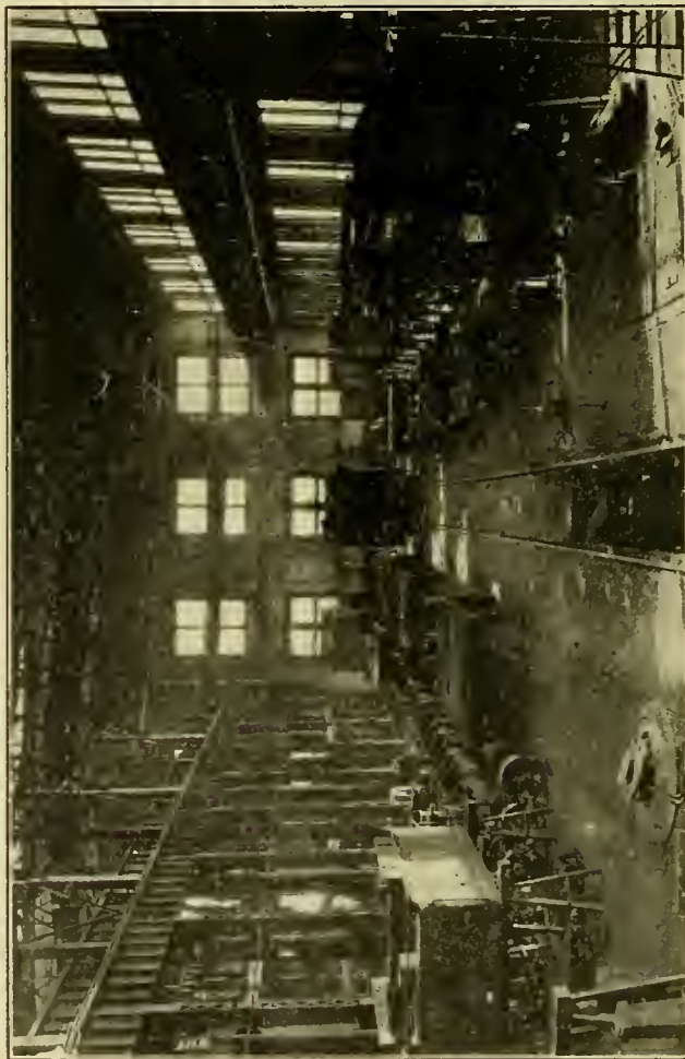
VIEW TAKEN FROM POINT C SHOWING THE TANK REPAIR SECTION. TANKS ARE REPAIRED ON ONE PIT; THE UNDER-FRAMES BETWEEN THE PITS AND THE TRUCK ON THE PIT NEXT TO THE BOILER SHOP.
