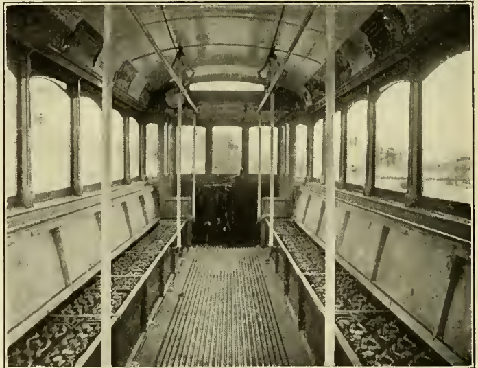
INTERIOR SHOWING STORAGE BATTERIES UNDER THE SEATS.
