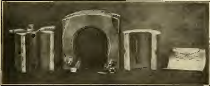
DRIVING BOX WITH REMOVABLE BRASS DISMANTLED.
