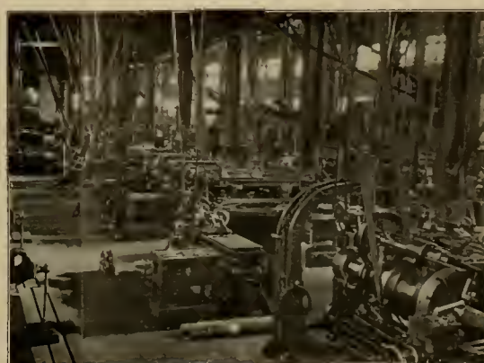
VIEW TAKEN FROM POINT E, SHOWING PART OF THE TOOLS DEVOTED TO ROD WORK. THIS IS UNDER THE BALCONY AND THE DRUMLEY AIR HOISTS ARE INDISTINCTLY SHOWN. ONE OF THE TILTHORNES TO THE TOOL ROOM WILL BE NOTICED ON ONE OF THE COLUMNS IN THE CENTRE DISTANCE.
