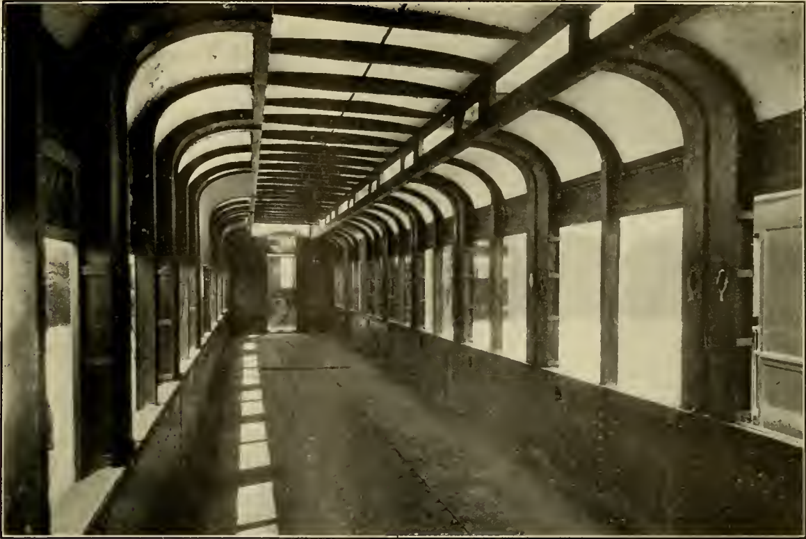
VIEW OF FRAMING FOR SLEEPING CAR.
