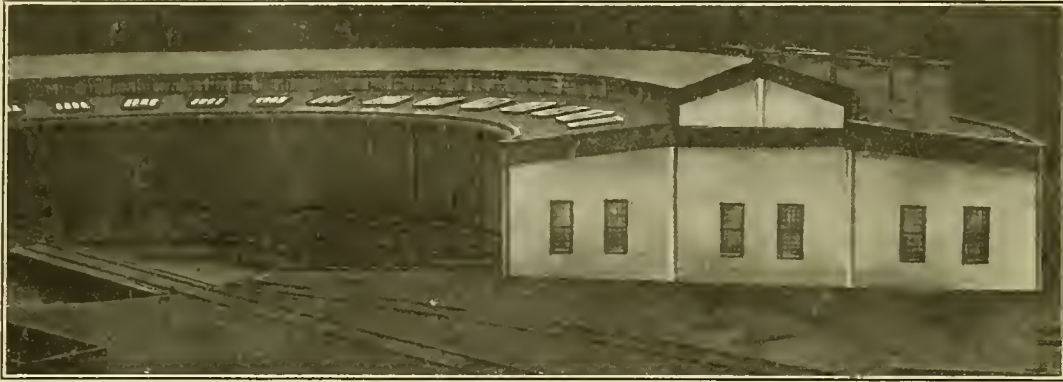
GENERAL VIEW OF THE REINFORCED CONCRETE ENGINE HOUSE AT OAK HILL—UNION RAILROAD.
