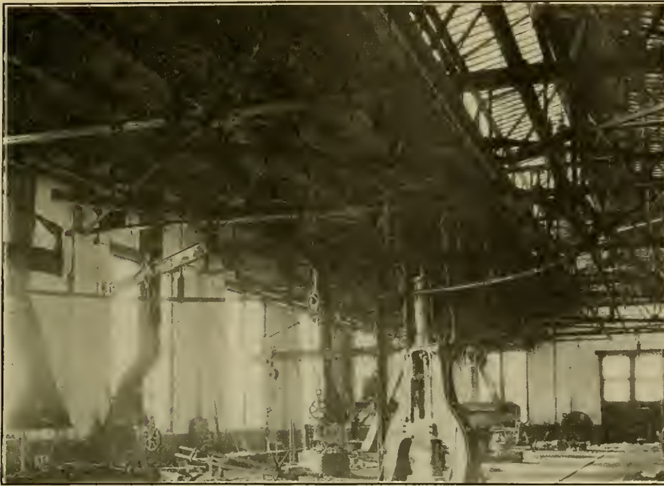
VIEW TAKEN FROM POINT I SHOWING A SECTION OF THE BLACKSMITH'S SHOP. THE CRANE COVERING A FULL CIRCLE, IS SUPPORTED ENTIRELY FROM THE ROOF AND SERVES A LARGE HAMMER, LARGE FORGE AND FACE PLATE AND TWO TRACKS. THE EXCELLENT OVERHEAD LIGHTING IS EVIDENT IN THIS PICTURE.
