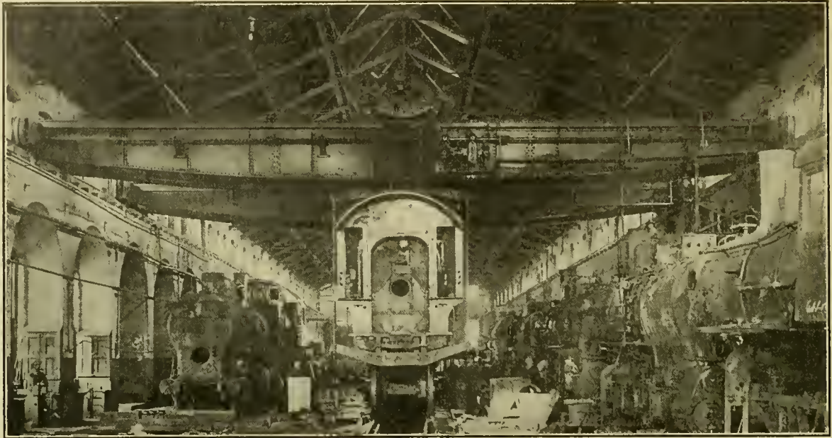
VIEW OF TWO 40-TON CRANES WHEELING A LOCOMOTIVE IN THE ROANOKE SHOPS OF THE NORFOLK & WESTERN RAILROAD.
