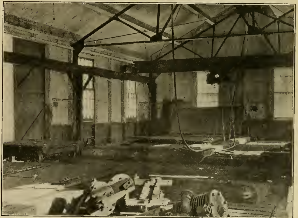
VIEW SHOWING THE INTERIOR OF THE CLEANING HOUSE. THE TRAVELING AIR HOIST, LARGE SIZE OF THE TANKS AND DRAINING PLATFORM, AS WELL AS THE STEEL FRAME WORK OF THE BUILDING, ARE WELL ILLUSTRATED BY THIS VIEW. THE HEAVY DOORS COVERING THE VATS ARE HANDLED BY THE HOIST.
