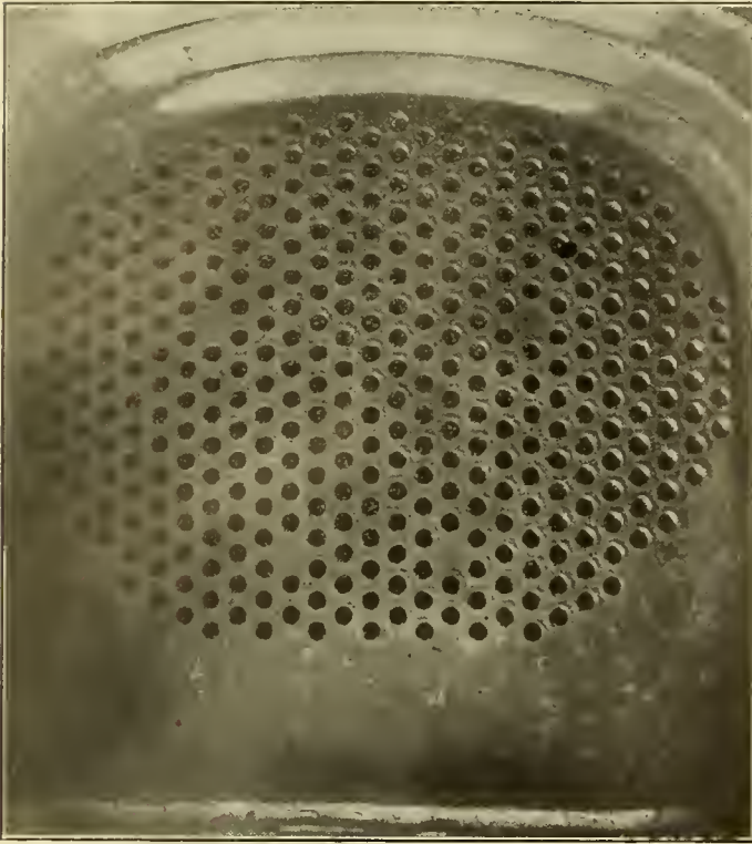
INTERIOR OF FIREBOX AFTER LOW WATER TEST. THE TUBES ARE WELDED IN THE SHEET BY THE AUTOGENEOUS PROCESS.
