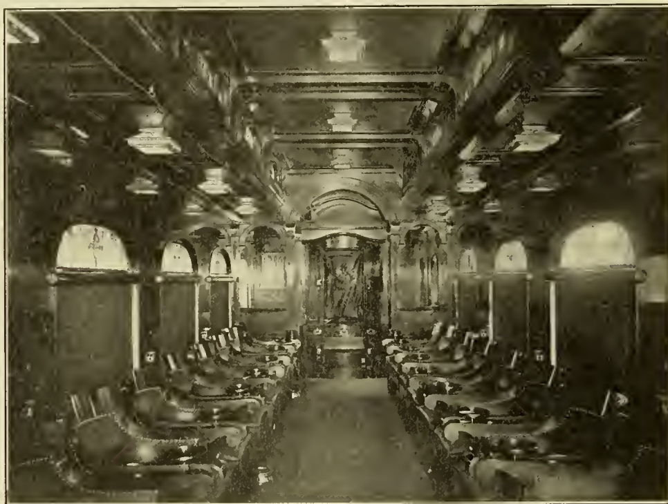
VIEW SHOWING THE HANDSOME INTERIOR OF THE SMOKING ROOM.
