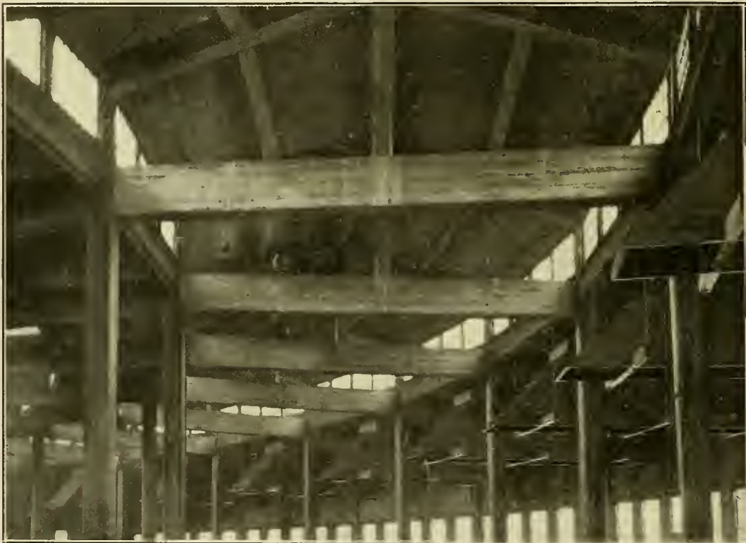
INTERIOR OF OAK HILL ENGINE HOUSE SHOWING ROOF BEAMS AND SMOKE JACKS.
