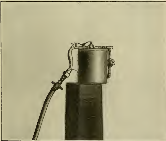
PAINT SPRAYER FOR PAINTING FRONT ENDS—LAKE SHORE & MICHIGAN SOUTHERN RAILWAY.
