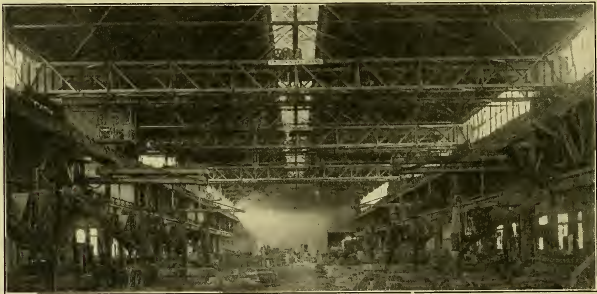
GENERAL VIEW OF THE FOUNDRY AT THE ROANOKE SHOPS OF THE NORFOLK & WESTERN RAILROAD. SEVEN NILES CRANES ARE SHOWN IN THIS ILLUSTRATION. THREE ARE 15-TON CAPACITY, HAVING LATTICE WORK GIRDERS; THE OTHER FOUR ARE OF THE WALL TYPE.
