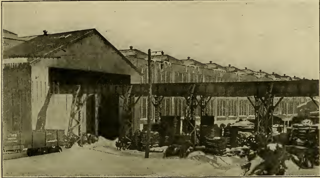
VIEW SHOWING THE TIRE HOUSE AND STORAGE YARD. WHEEL CENTRES AND OTHER HEAVY CASTINGS ARE UNLOADED FROM THE CARS TO THE CONCRETE PLATFORMS UNDERNEATH THE CRANE, WHERE THEY ARE STORED UNTIL NEEDED. ALL REMOVING AND APPLYING OF TIRES IS DONE IN THE BUILDING SHOWN AT THE LEFT.
