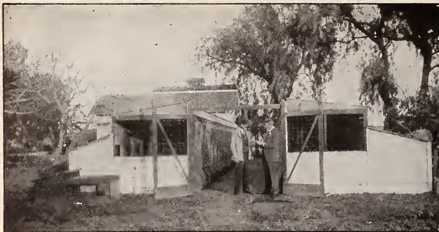
UNIQUE COCKEREL HOUSE BUILT AND OWNED BY J. V. McCONNELL
