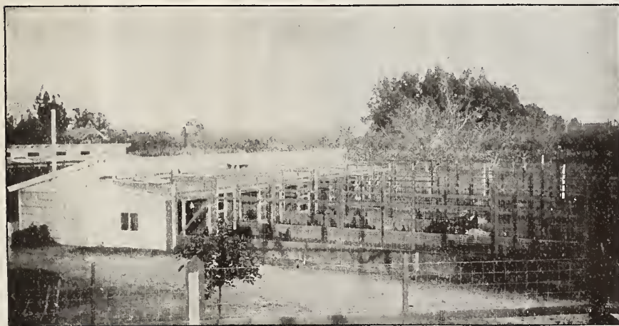
VIEW OF SIX-PEN BREEDING HOUSE AND BROODING HOUSE FROM RESIDENCE SIDE
