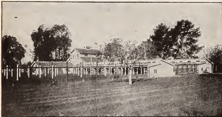
VIEW OF McCONNELL SIX-PEN BREEDING HOUSE, ETC., FROM FIELD
