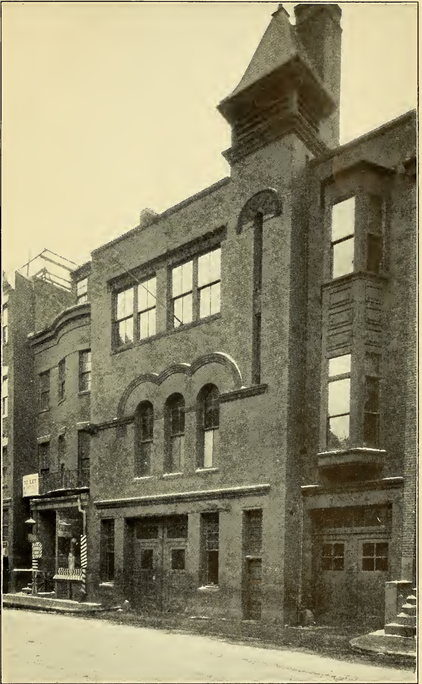
OLD QUARTERS OF ENGINE COMPANY 6, LEVERETT STREET, REPLACED BY NEW FIRE STATION IN BOWDOIN SQUARE.
