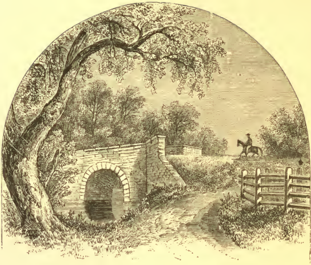
THE STONE BRIDGE.
