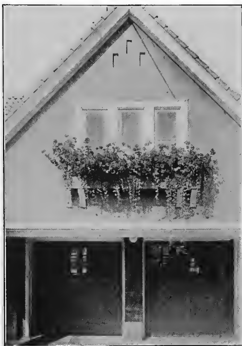
Concrete window box as an integral part of the building; in this case a garage
