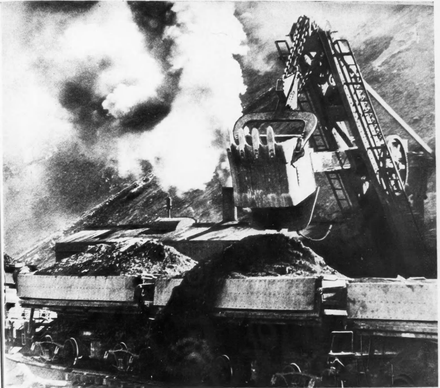
A steam shovel in action at Jerome, Arizona, on United Verde Copper Company's ground
