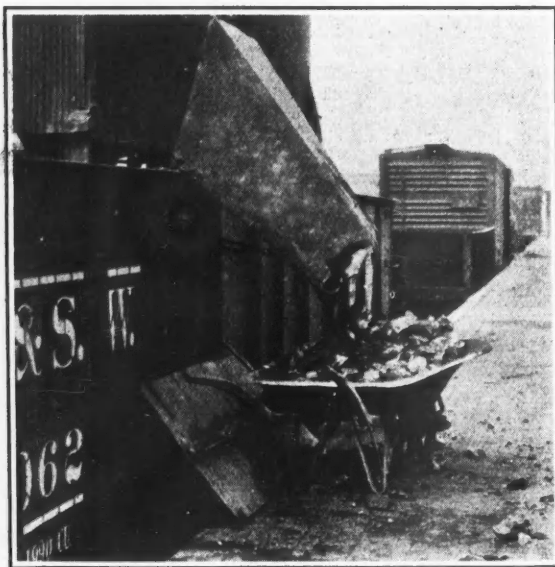
Unloading hopper for non-dumping railroad cars
