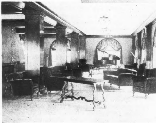
A corner of the mezzanine above the lounge. It serves as a reading, writing and music room
