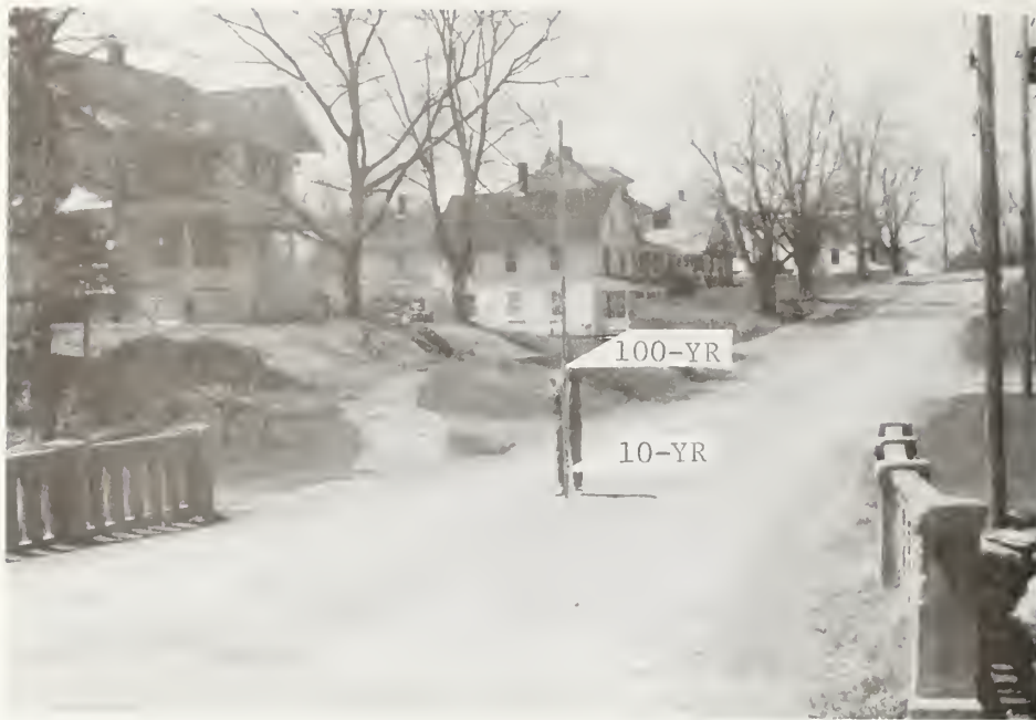
Pearce Brook, Green Street, cross section 210B. The 100-year flood is estimated to be at elevation 354.1 feet NGVD or 5.3 feet above the road. (SCS photo)
