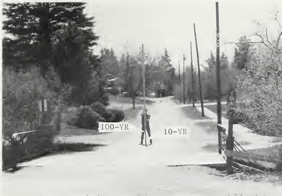
Pearce Brook, Brook Street, cross section 215B. The 100-year flood is estimated to be at elevation 358.4 feet NGVD or 2.0 feet above the road. (SCS photo)
