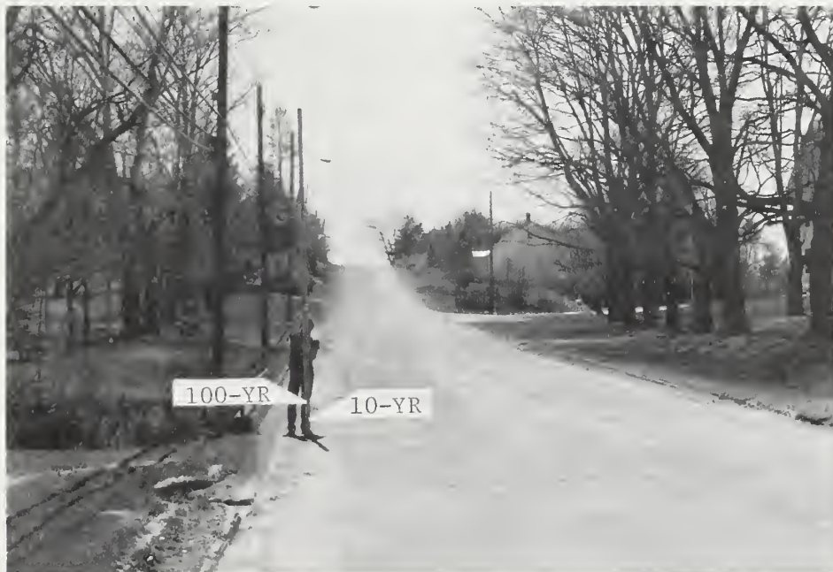
Pearce Brook, Court Street (U.S. Route 1), cross section 218B. The 100-year flood is estimated to be at elevation 366.6 feet NGVD or 1.6 feet above the road. (SCS photo)
