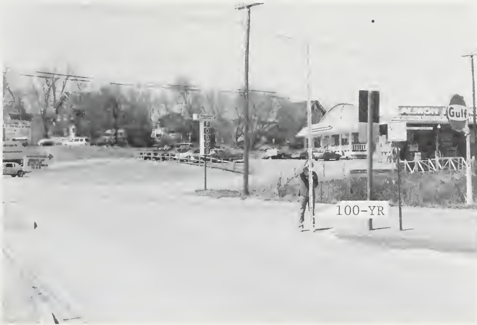
Pearce Brook, Bangor Street (U.S. Route 2A) at its intersection with Military Street, cross section 202B. A 100-year flood would reach an estimated elevation of 347.4 feet NGVD or 1.3 feet above the road at this busy intersection. (SCS photo)
