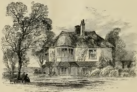
Barley Wood, Residence of Hannah More.
