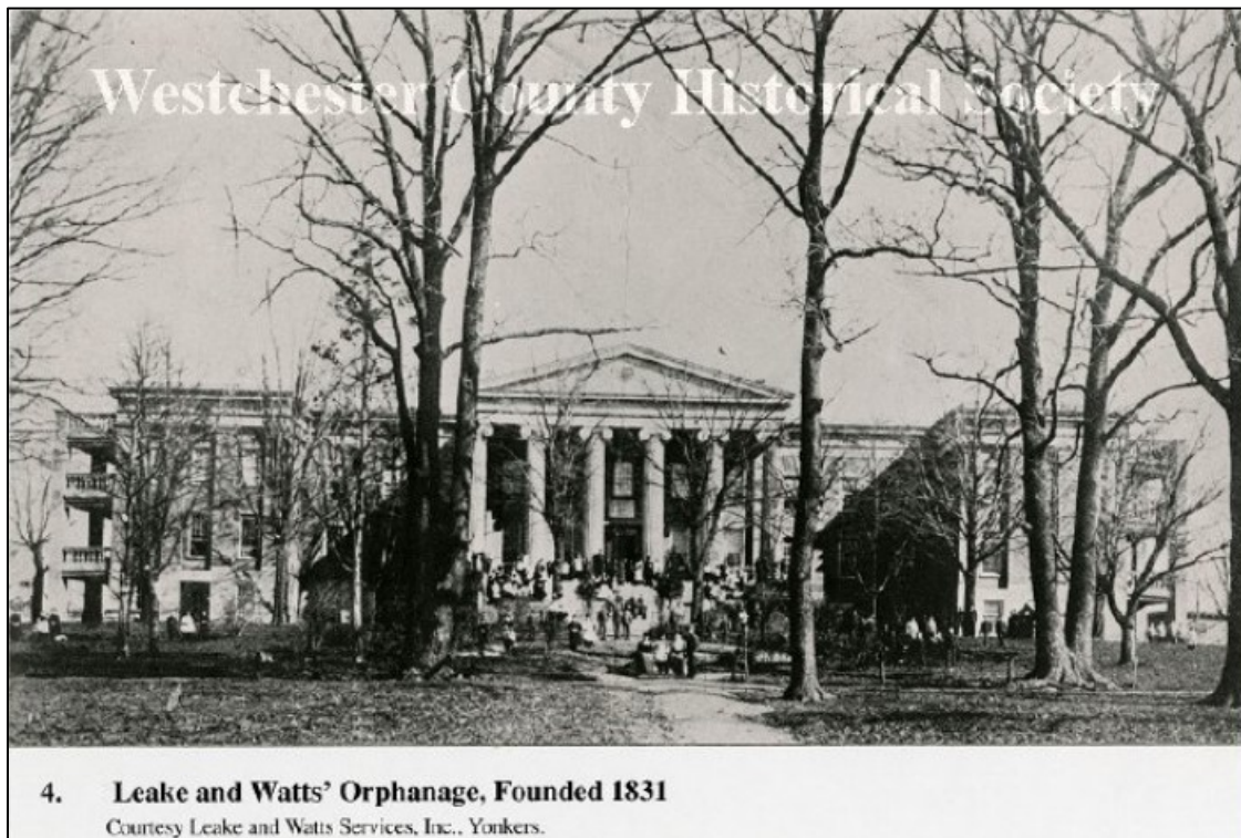
Leake and Watts' Orphan House: date unknown.
