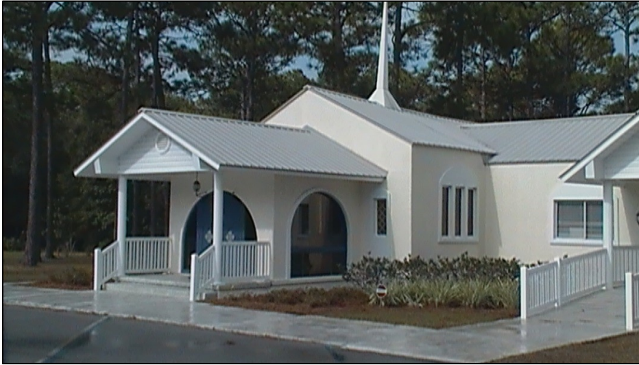
Jules' original church in Panama City at new location. The building was moved from its original location to here. New addition on right.
