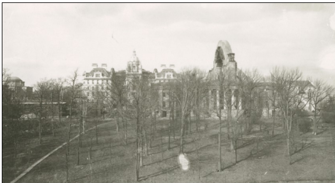
Leake and Watts' Orphan House: date unknown.
