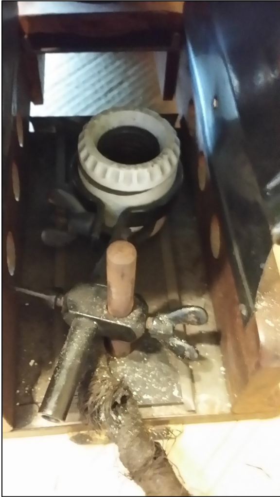
Lantern: Electrical work was done.
