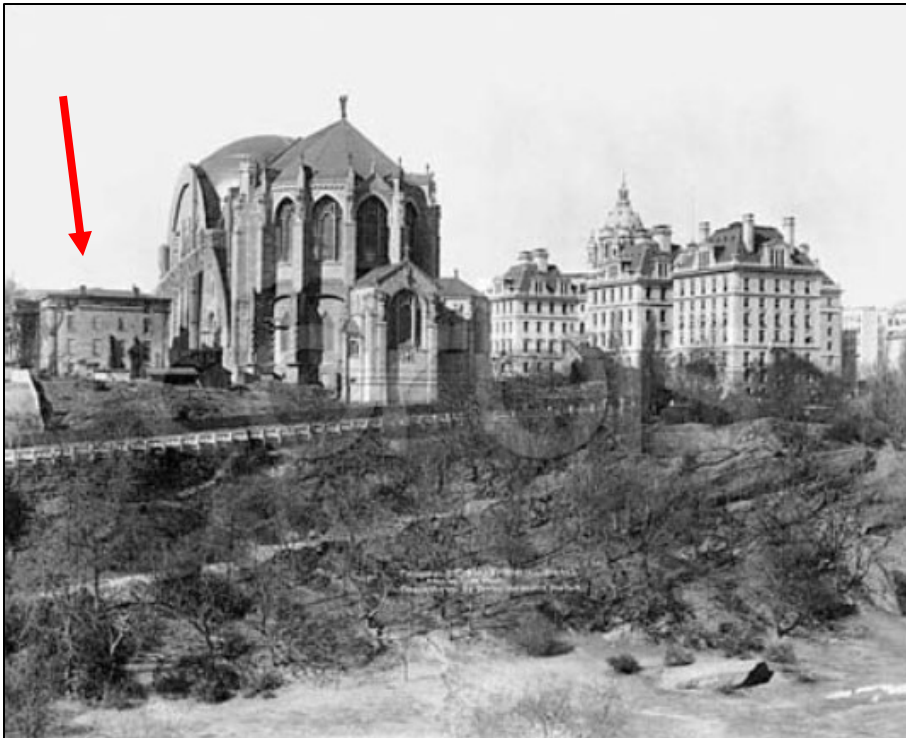
Leake and Watts building below red arrow.
