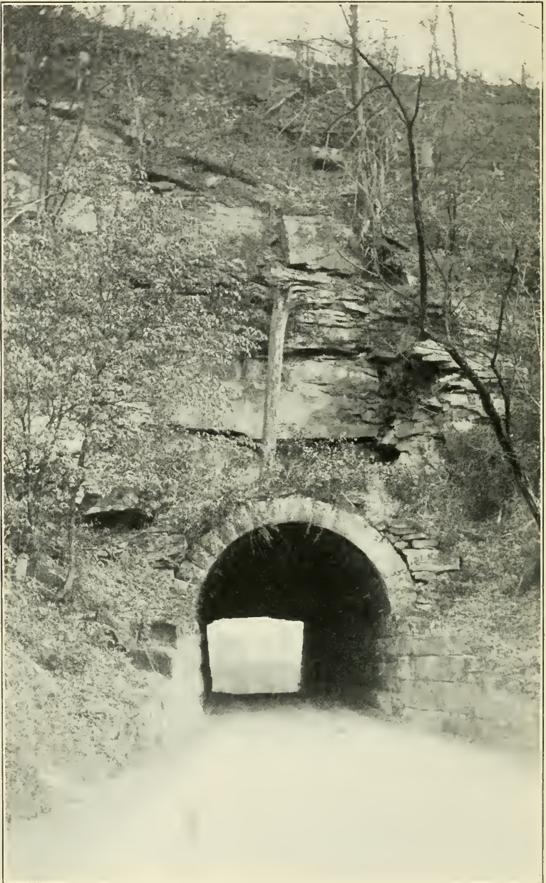
Plate III.—Wellsburg-Bethany Turnpike Tunnel, With Morgantown Sandstone Above, Brooke County.
