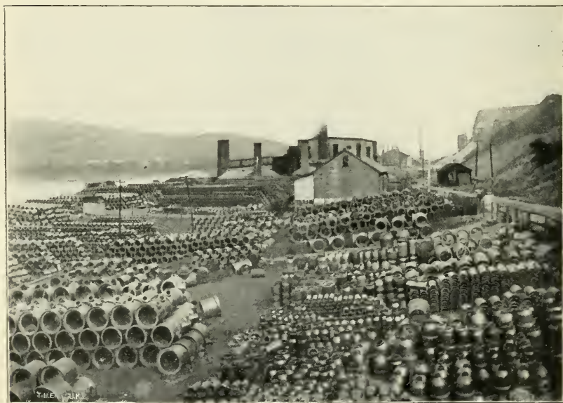
Plate XVI.—b. Clifton Sewer Pipe Yard, New Cumberland, Hancock County.
