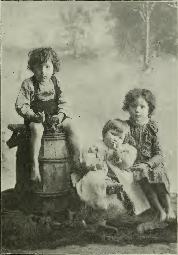
FROM VERY BAD SURROUNDINGS.
