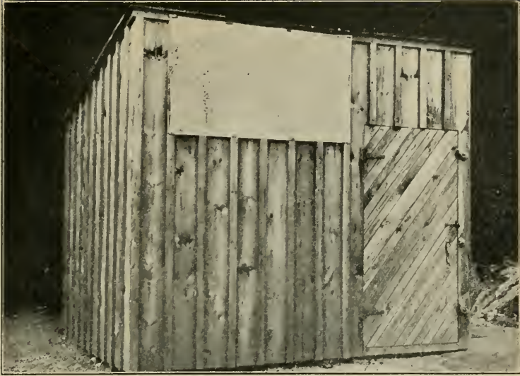
Fig. 1. Fumigation house at the Agricultural College, Guelph, size, 8 x 10 x 7½; two doors, front and back; wooden buttons on door. The earth was banked well around the outside. Cost: dressed lumber, $16.00; hardware, $2.55; labor, $5.00; total, $23.55. By using undressed lumber the cost would be $4.00 less. (The photo was taken before the earth was banked up.)
