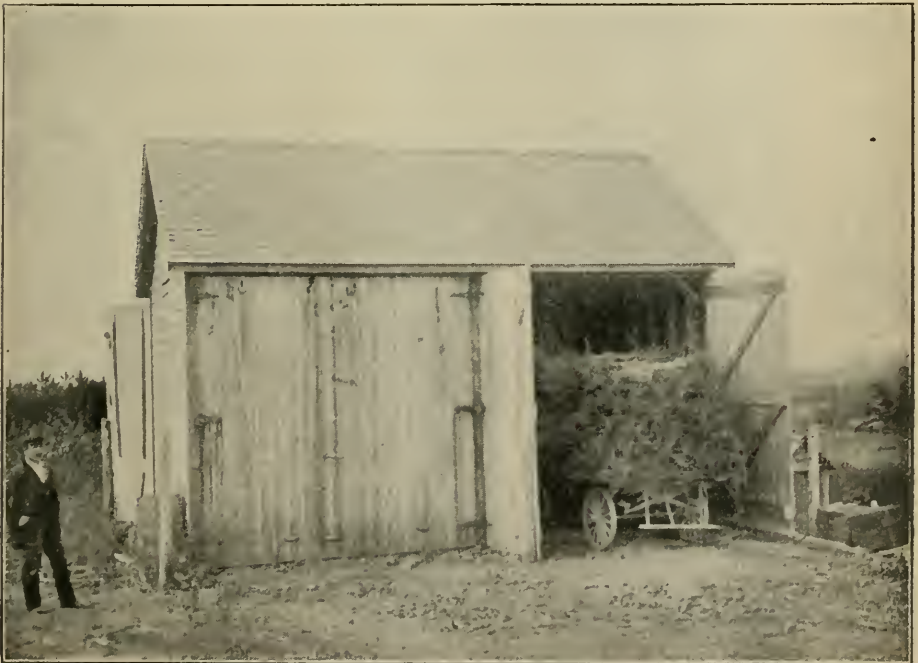
Fig. 2. Fumigation house of Mr. E. D. Smith, Winona. This is a double house of two large compartments. The stock is fumigated on the wagon. Such a house is suitable for large nurseries only.
