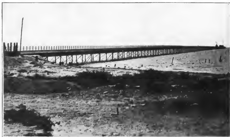
STEEL PILE PIER OF THE BARRANQUILLA RAILWAY AND PIER COMPANY (LIMITED), AT PUERTO COLOMBIA, THE ACTUAL SEAPORT FOR BARRANQUILLA, COLOMBIA.
