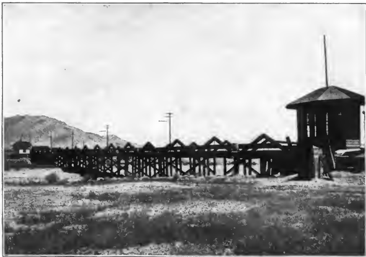
THE INTERNATIONAL BRIDGE OVER THE RIO GRANDE, OR THE RIO BRAVO.
