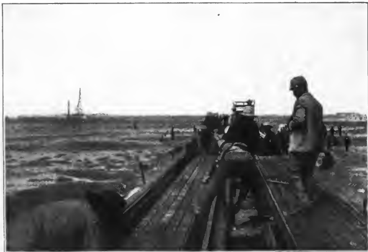
TRACK LAYING NEAR ORURO.
