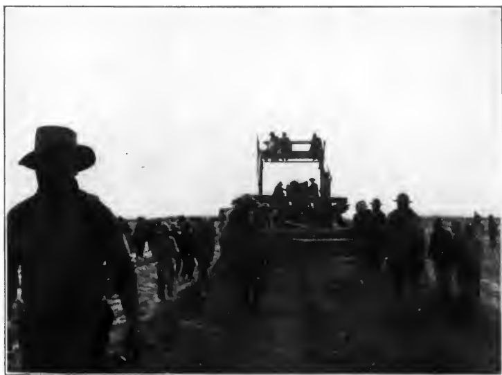
TRACK LAYING INTO ORURO.
