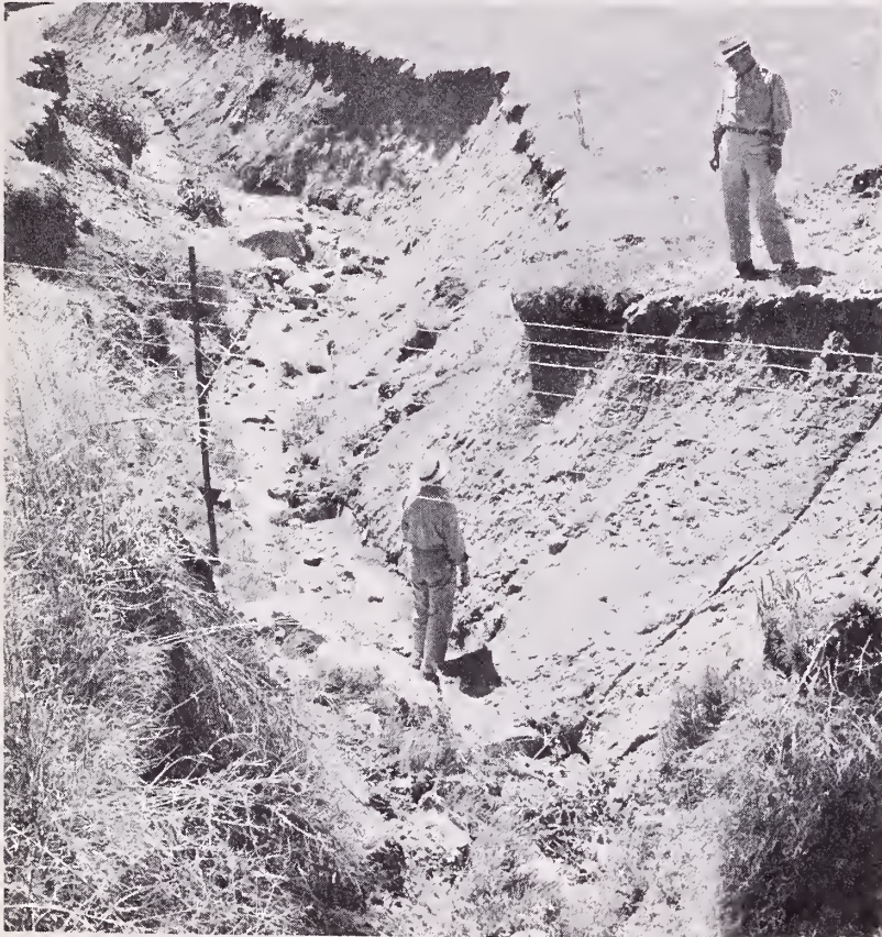
Tons of valuable soil have been washed from the pasture at the left leaving a meandering gully which has isolated a portion of the land from both machinery and livestock. SD 517
