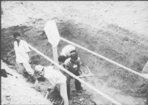
Workers dig a water collection pit on the embassy compound.
