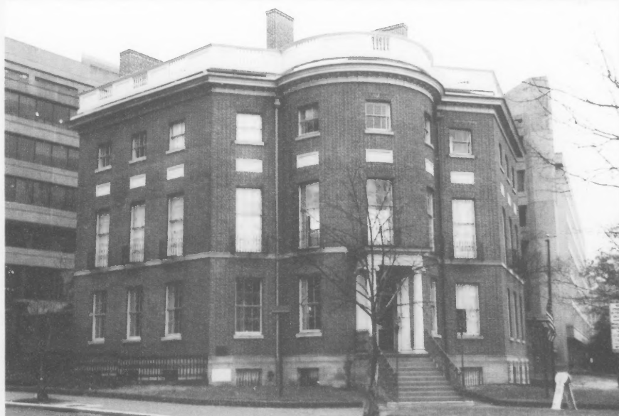
Above: The Octagon House on New York Avenue was a Department annex during World War II. Below: The George C. Marshall wing of Main State was once known as New State. Surrounded by a construction fence, it is under renovation.
