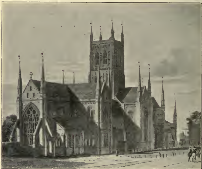
THE EXTERIOR, FROM THE NORTH-EAST, BEFORE RESTORATION. (From Wild.)
