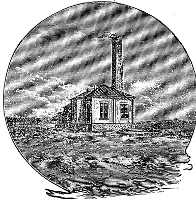
WATER WORKS PUMPING STATION.
