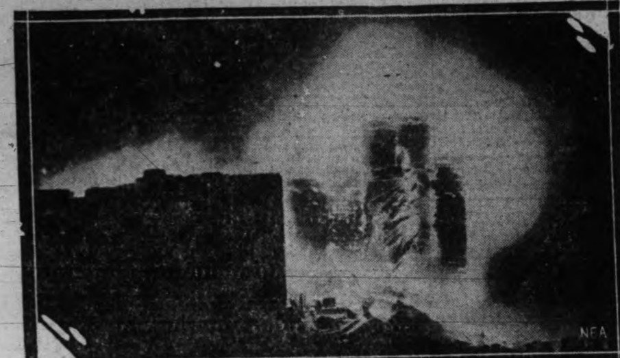
A MILLION-DOLLAR FIRE AT ITS HEIGHT —Six hundred thousand bushels of grain were destroyed and the steel tow barge Alexander Maitland with 150,000 bushels of barley in her hold was badly damaged in an early morning fire in the Grand Trunk elevator at Port Huron, Mich. This picture was taken while the fire was at its height, just after the elevator's roof fell, showering burning brands over a two-mile area. The loss is estimated at $1,000,000.
