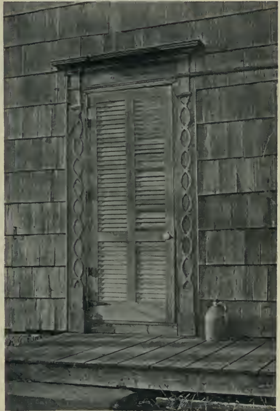
Doorway Detail. THE ANNA HALSEY HOUSE, WATERMILL, LONG ISLAND.
