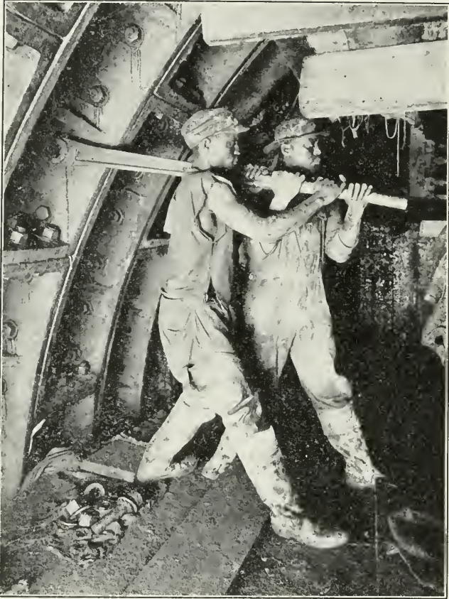
TIGHTENING BOLTS IN TUNNEL LINING, NORTH TUNNEL, BY MEANS OF RATCHET WRENCH. EACH BOLT WEIGHS 10 POUNDS
