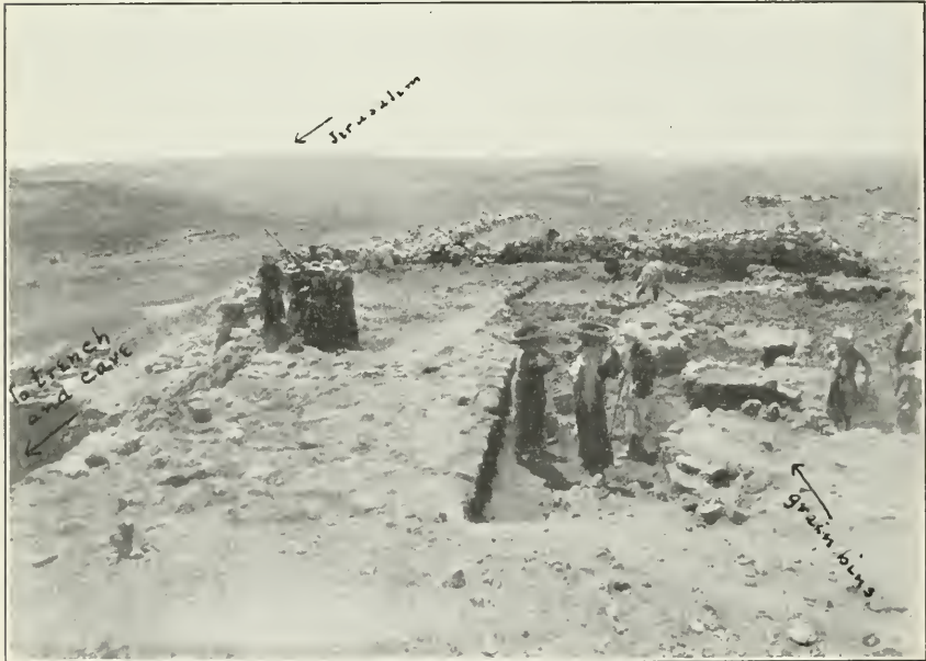
2. TOP OF CITY WALL ABOVE THE TRENCH AND CAVE ON THE EASTERN SLOPE
