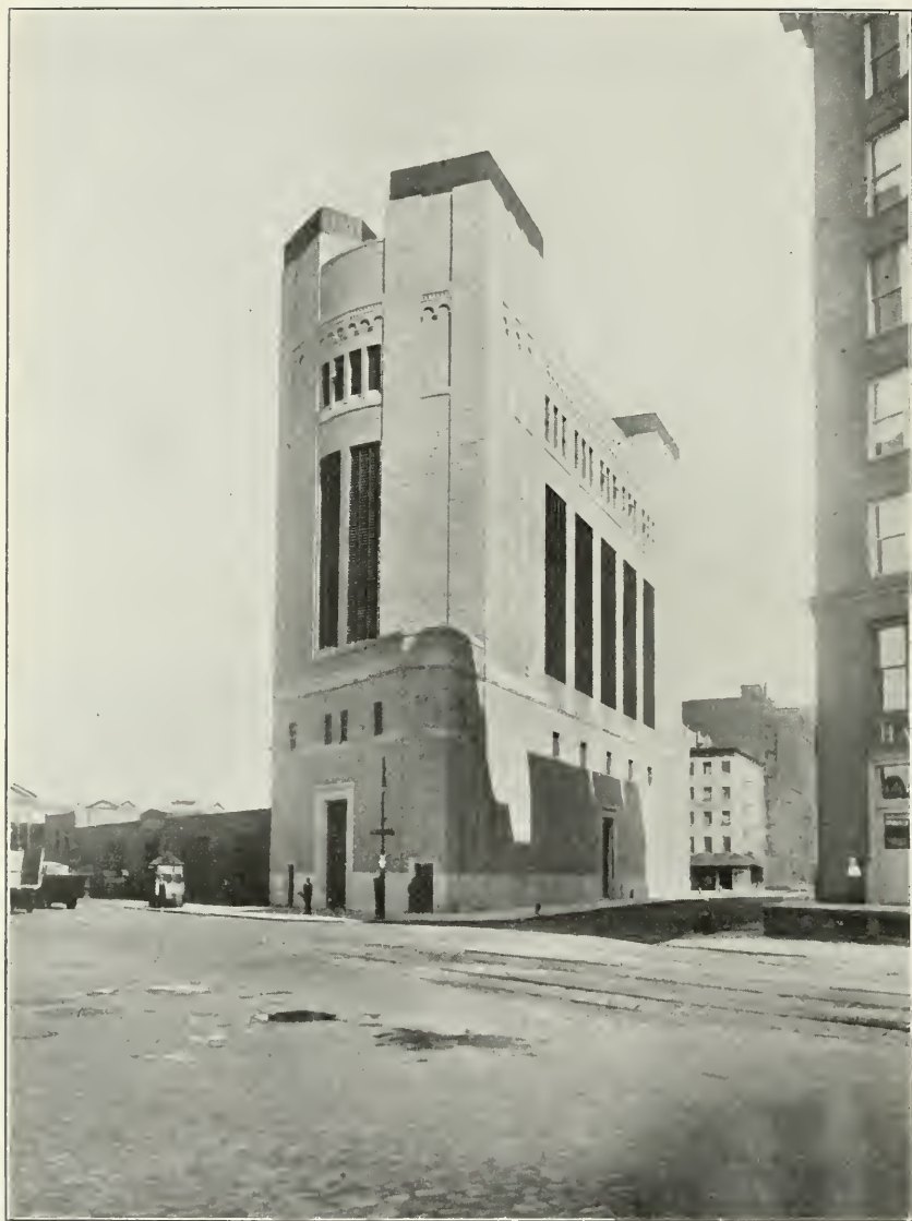
LAND VENTILATION BUILDING
