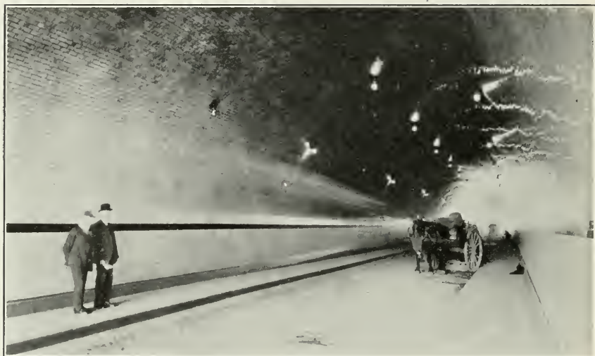
REST AND REFRESHMENT IN ROTHERHITHE TUNNEL, RIVER THAMES, LONDON, ENGLAND
