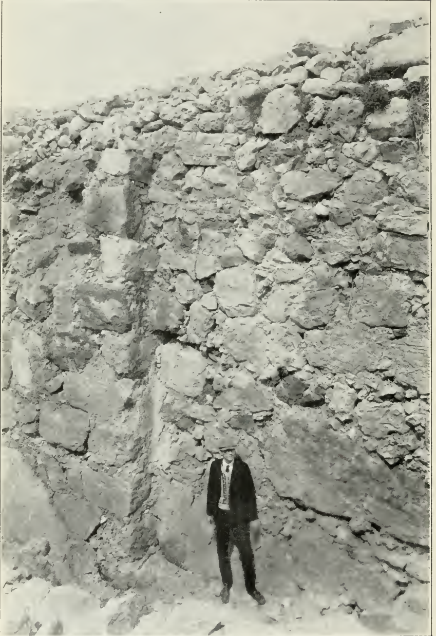
MASONRY OF CITY WALL AT THE SOUTH END, OUTER FACE; THICKNESS 20 FEET
