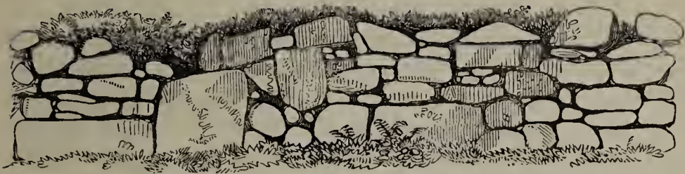
Chûn Castle. Masonry of outer Wall.
