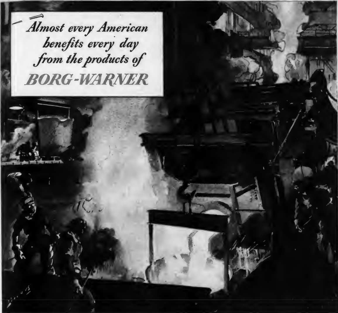
"THE WEDDING OF THE STEELS" at the Ingersoll plant, New Castle, Indiana. James Sessions catches the tense moment when soft center steel is poured in the final step before it joins with stainless steel to form "IngAclad." A similar process is used in making soft center plow mold boards. Alloy steels for saws and for the chemical and food industries come from this great Borg-Warner mill.
