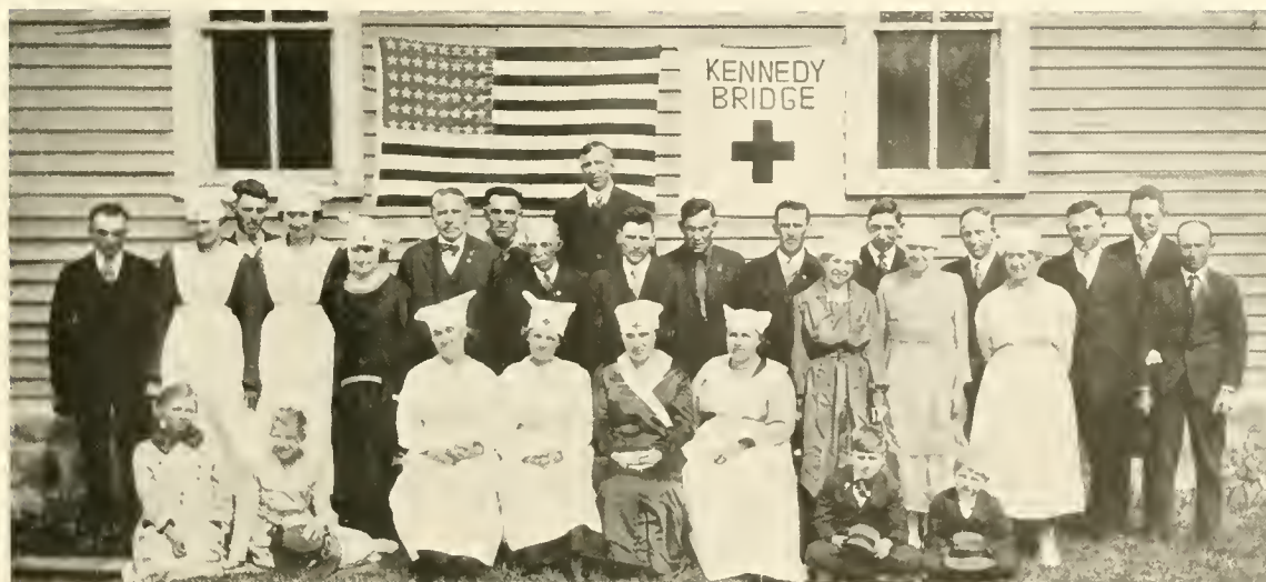
KENNEDY BRIDGE RED CROSS BRANCH
