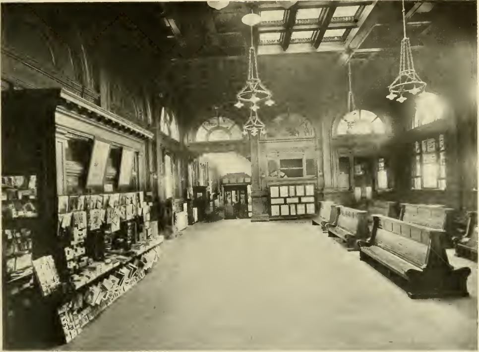
INTERIOR WAITING-ROOM, WEST 23D STREET STATION
