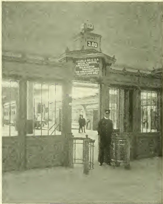
GATE TO TRAIN SHEDS
