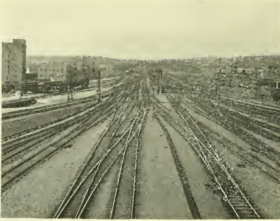
TRACKS LOOKING FROM STATION
