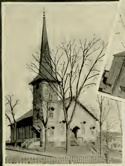
Photos by Wendt, Boonton. Presbyterian Church
