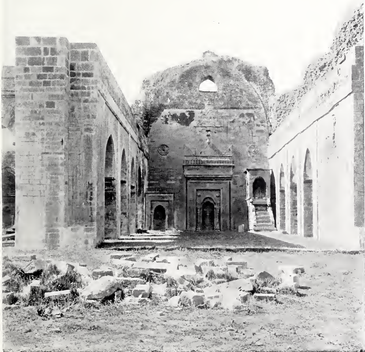
ĀDĪNAH MOSQUE, CENTRAL CHAMBER IN WESTERN CORRIDOR
