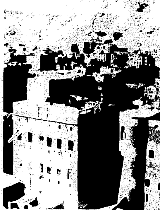
FIGURE 8. Most highland towns are congested. They consist of closely spaced multistory buildings of sun-dried clay and mud or stone. Roofs are flat and surmounted by parapets, and streets are narrow and unsurfaced. This is Tarim, which lies in Wadi Hadramawt. (U/OU)
