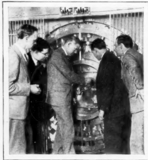
Interior View of Vault, Showing Handle That Unlocks Door from Inside
