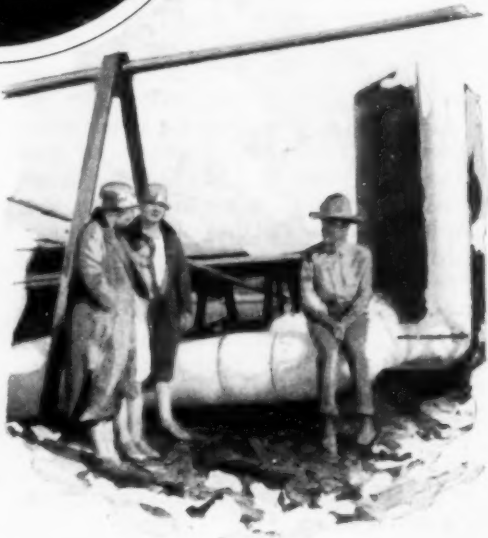
The Freak Well, Frozen Valves, and a Cool Seat for One of the Workmen While Resting
