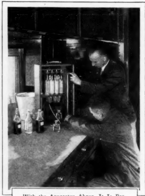
With the Apparatus Above, It Is Possible, by Analyzing a Sample of Air, to Tell Whether Fire Is Raging Underground, or Poison Gas Is Present in Dangerous Amounts
