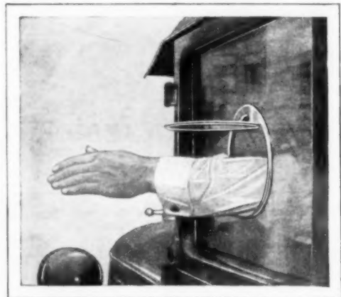
Hinged Section in Auto Door for Making Arm Signals; Opening Also Is Aid to Ventilation
