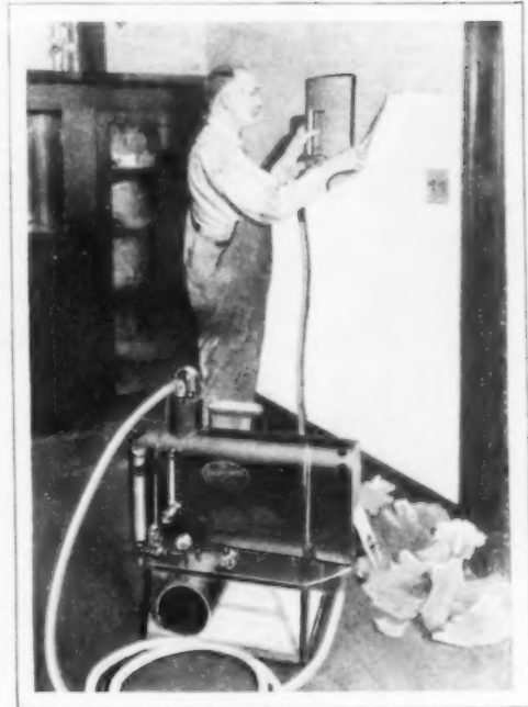
Removing Old Wall Paper with the Portable Steaming Outfit, Which Also Cleans the Wall
