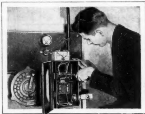
Tightening Switch-Box Connections; Condensers Are Shown Connected above the Box
