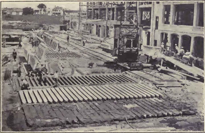
FIGURE 143. MANUFACTURING REINFORCED CONCRETE PILES.
