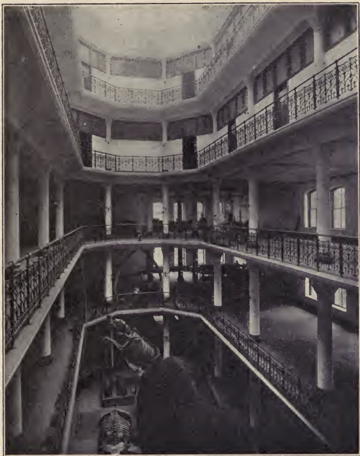
FIGURE 4. — ACADEMY OF SCIENCES, SAN FRANCISCO Reinforced Concrete Floors, Cast Iron Columns Erected by Ernest L. Ransome
