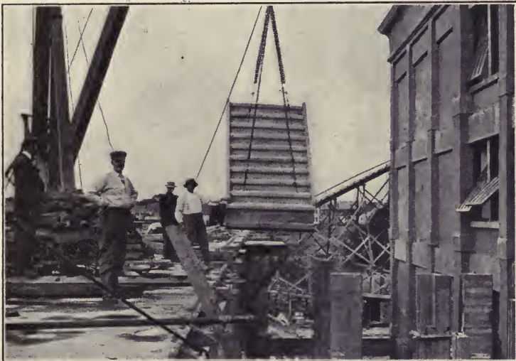
FIGURE 140. SETTING A FLIGHT OF STAIRS.
