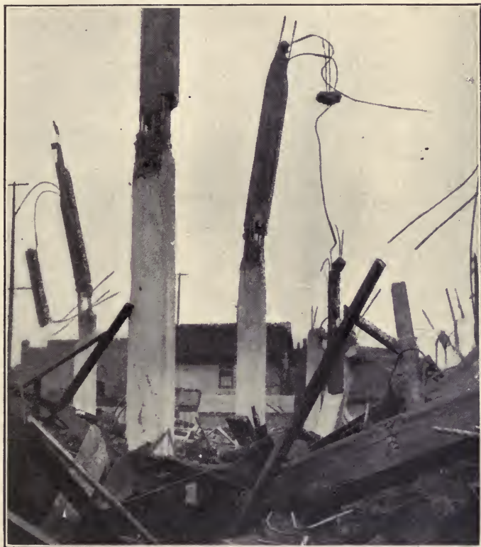
FIGURE 147. WRECK OF THE HENKE BUILDING IN CLEVELAND.
