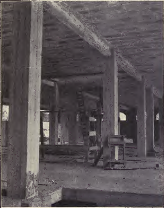
FIGURE 89. TILE CONCRETE CONSTRUCTION, READY FOR PLASTERER
