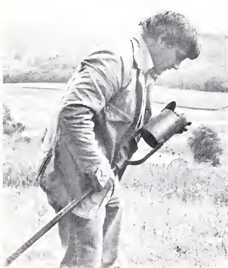
At left, Tim McCormick, OSSP specialist, uses a soil auger to test soil for depth, permeability, stoniness, and other characteristics that could affect sewage treatment.
