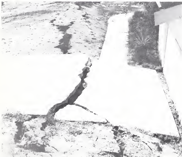
Driveway broken up—another of the problems caused by soil subsidence. Information in soil surveys can be used to avoid these problems.
