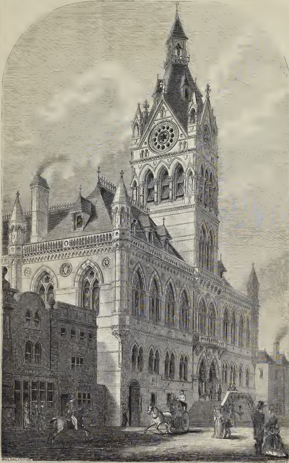
CHESTER TOWN-HALL.—MESSRS. LANYON, LYNN, & LANYON, ARCHITECTS.
