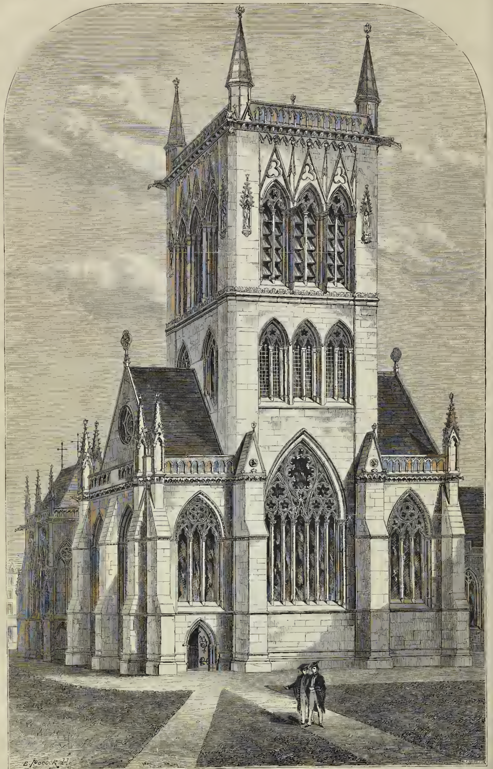
THE CHAPEL OF ST. JOHN'S COLLEGE, CAMBRIDGE: WEST FRONT. PROFESSOR G. G. SCOTT, R.A., ARCHITECT.
