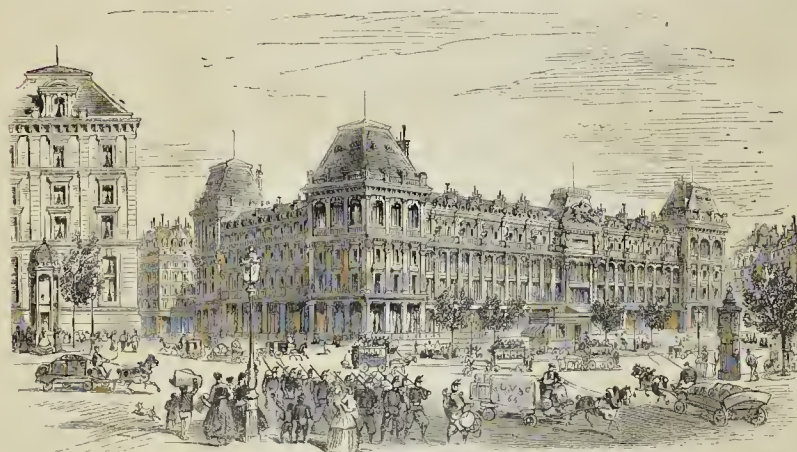
View on the Boulevards near the Chateau d'Eau.
