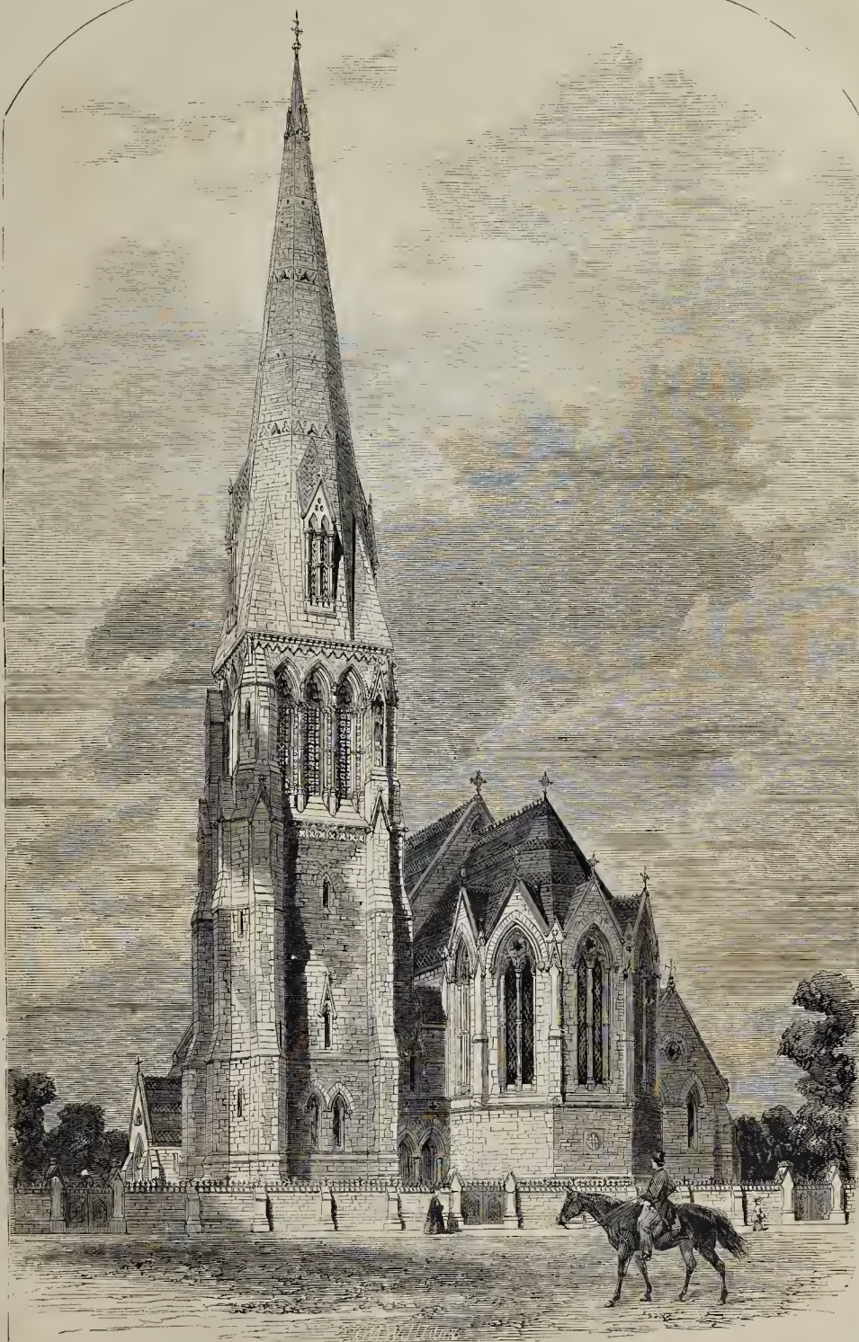
ST. MATTHEW'S CHURCH, UPPER CLAPTON, MIDDLESEX.—MR. FRANCIS T. DOLLMAN, ARCHITECT. [See p. 262, ante.]
