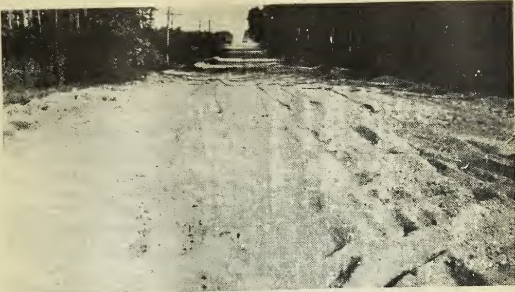
APPEARANCE OF THE ROAD AFTER SCARIFYING
