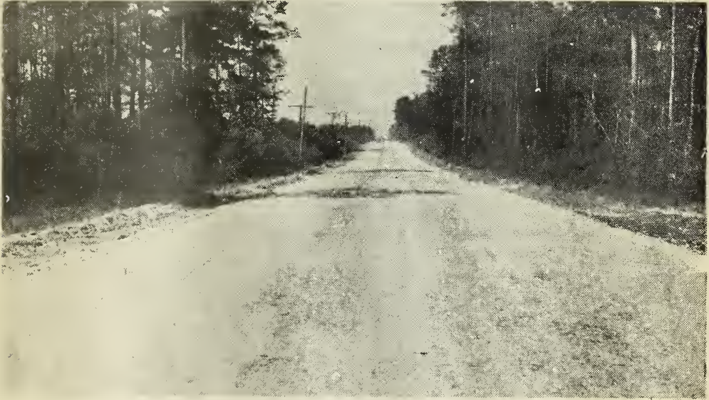
APPEARANCE OF THE DOUBLE SURFACE TREATMENT ON A MIXED-IN-PLACE BASE
