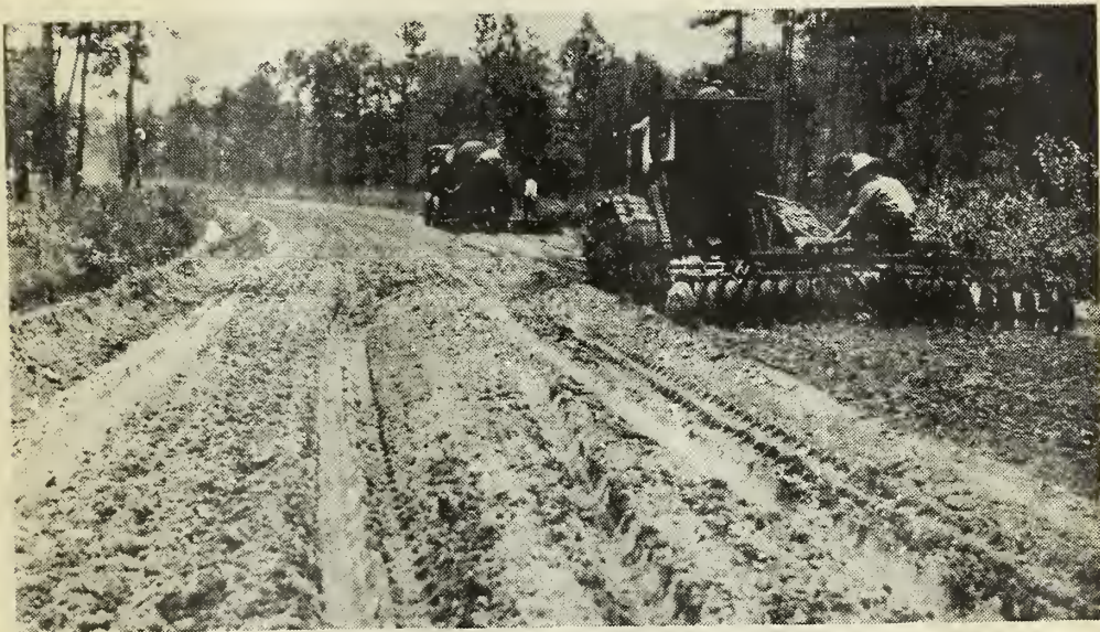
APPLYING BITUMINOUS MATERIAL AND DISCING
