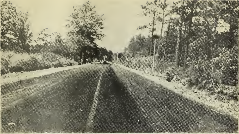
MIXING AND SHAPING WITH GRADER
