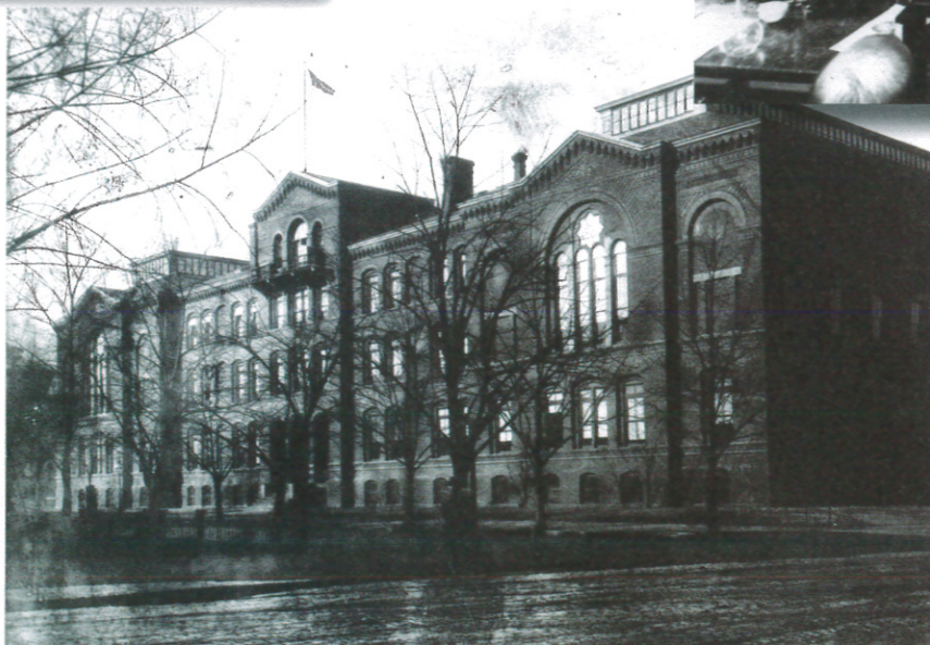
A photograph of the museum building following completion in 1887. The building became known as the “Old Red Brick.” (AMM 740)
