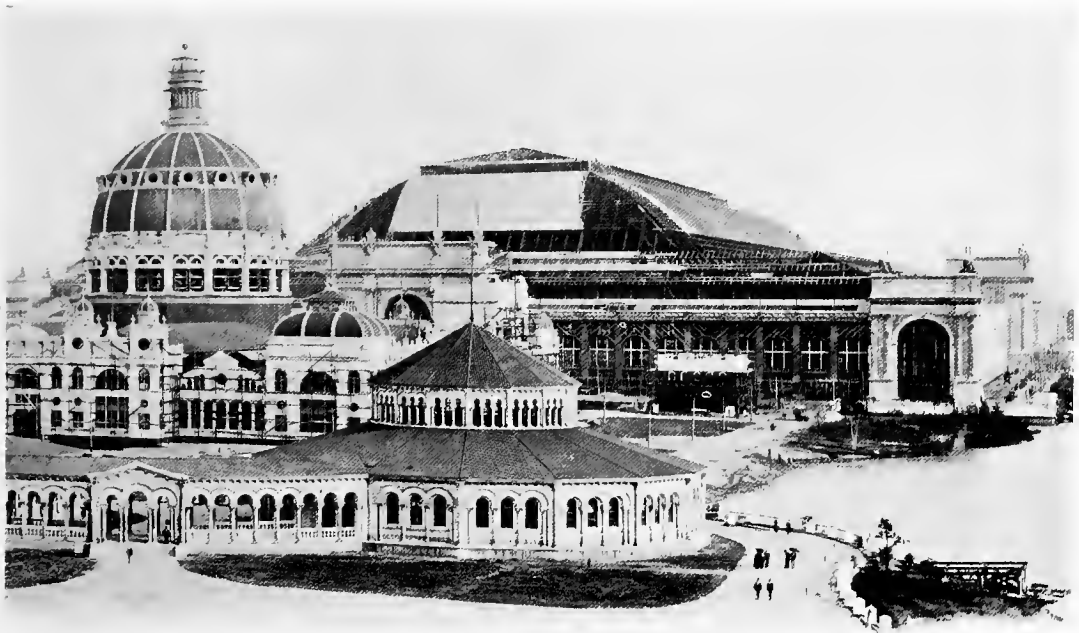
APPROACHING COMPLETION. LOOKING SOUTHEAST.
