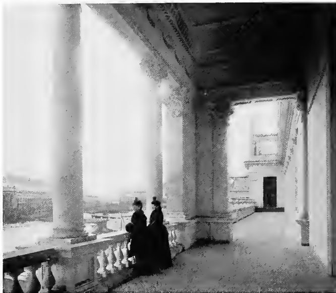
LOGGIA OF THE WOMAN'S BUILDING, looking eastward across the Wooded Island.
