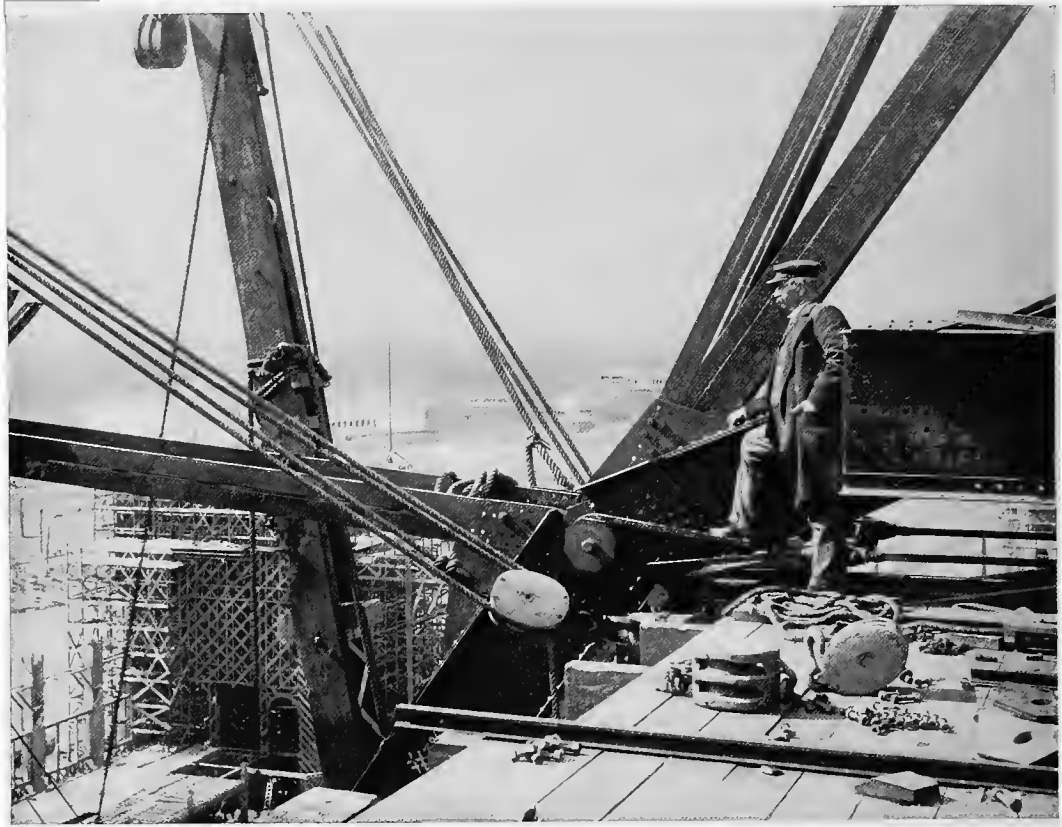
AN ARCH JOINT, 125 feet from the ground, in the Manufactures Building, April 10, 1892.
