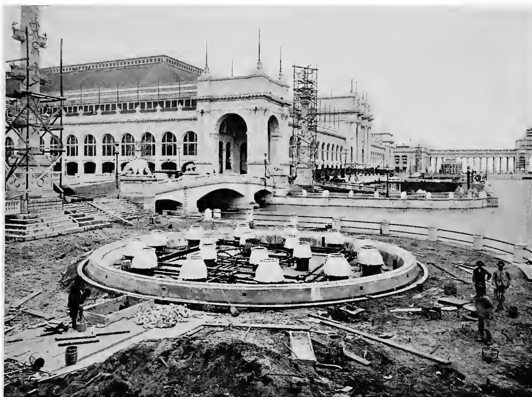
CONSTRUCTION OF THE NORTH ELECTRIC FOUNTAIN.
