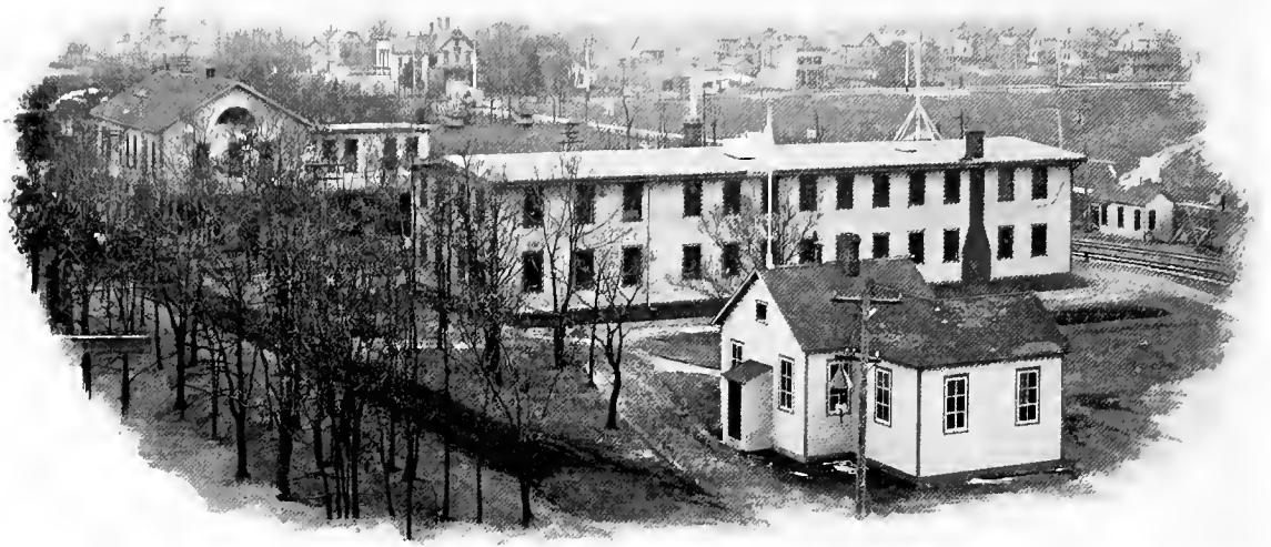
Temporary Offices and Hospital, February 5, 1892.
