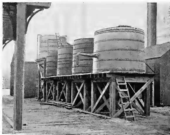
Tanks for purifying drinking-water.
