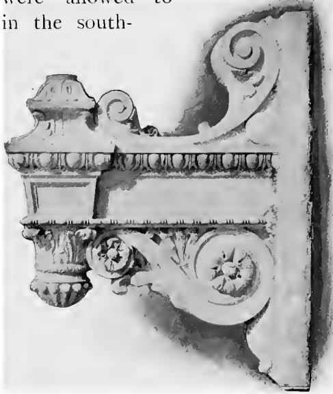
STAFF DETAIL FOR THE MANUFACTURES BUILDING.
