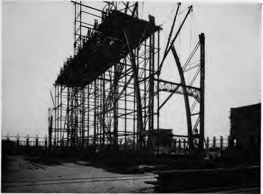
RAISING TWO ARCHES OF THE MANUFACTURES BUILDING, MARCH 26, 1892.
