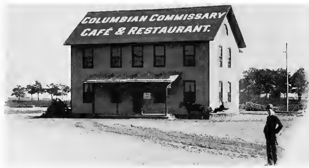
Commissary Building, October 12, 1891.
