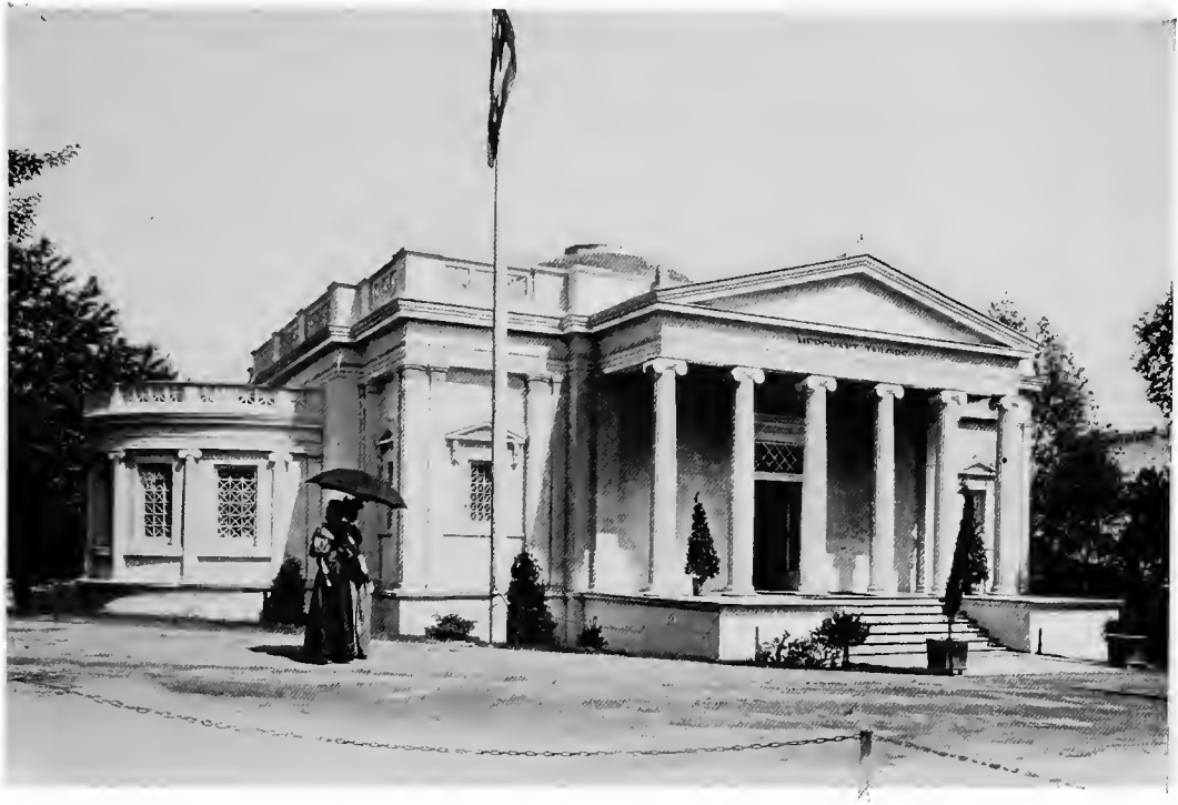
THE MERCHANT TAILORS' BUILDING.
