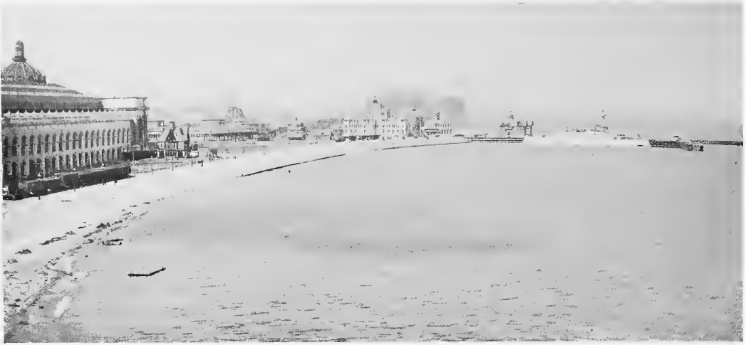
The Lake Front with the Buildings near Completion.
