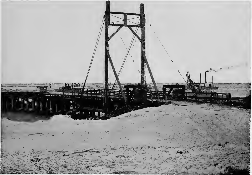
RAILROAD BRIDGE OVER THE GRAND CANAL, JULY 30, 1891.
