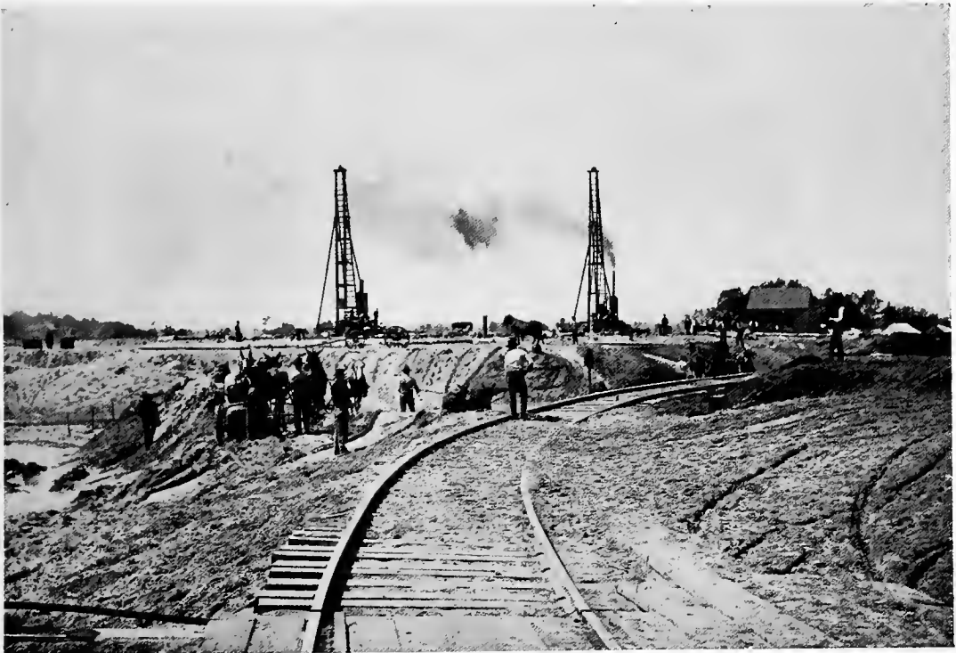
SITE OF THE ADMINISTRATION BUILDING, looking west, August 21, 1891.
