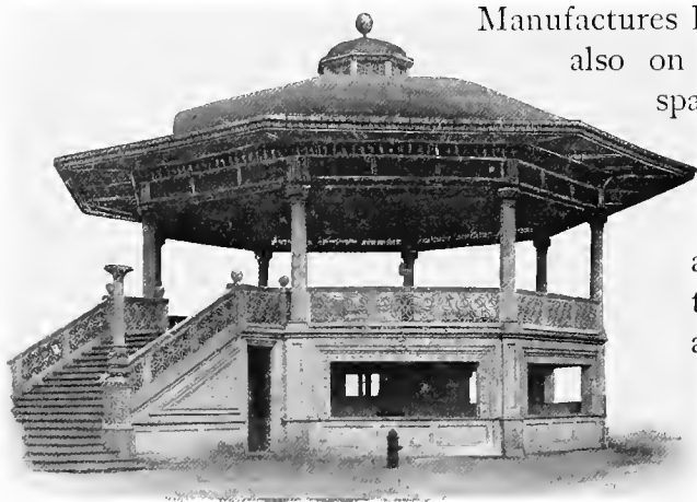
ONE OF THE BAND STANDS, Designed by Charles B. Atwood.
