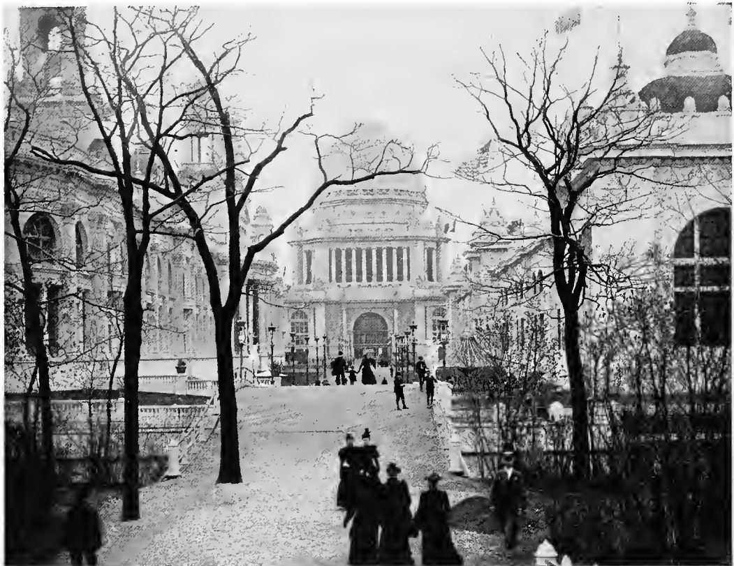
THE ADMINISTRATION BUILDING, from the Bridge to the Wooded Island.
