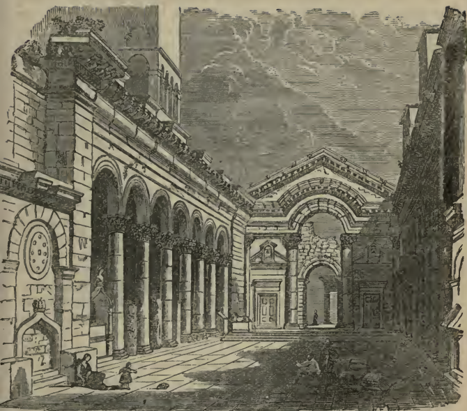
The Court-yard of Diocletian's Palace at Spalatro.
