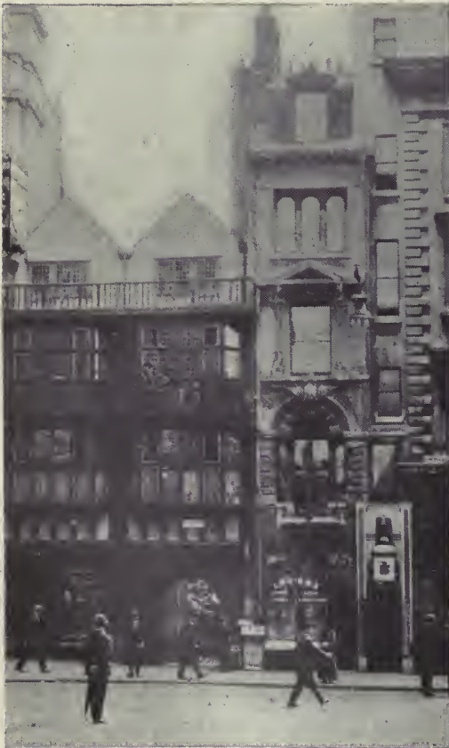
GROOM'S COFFEE HOUSE, FLEET STREET, LONDON
