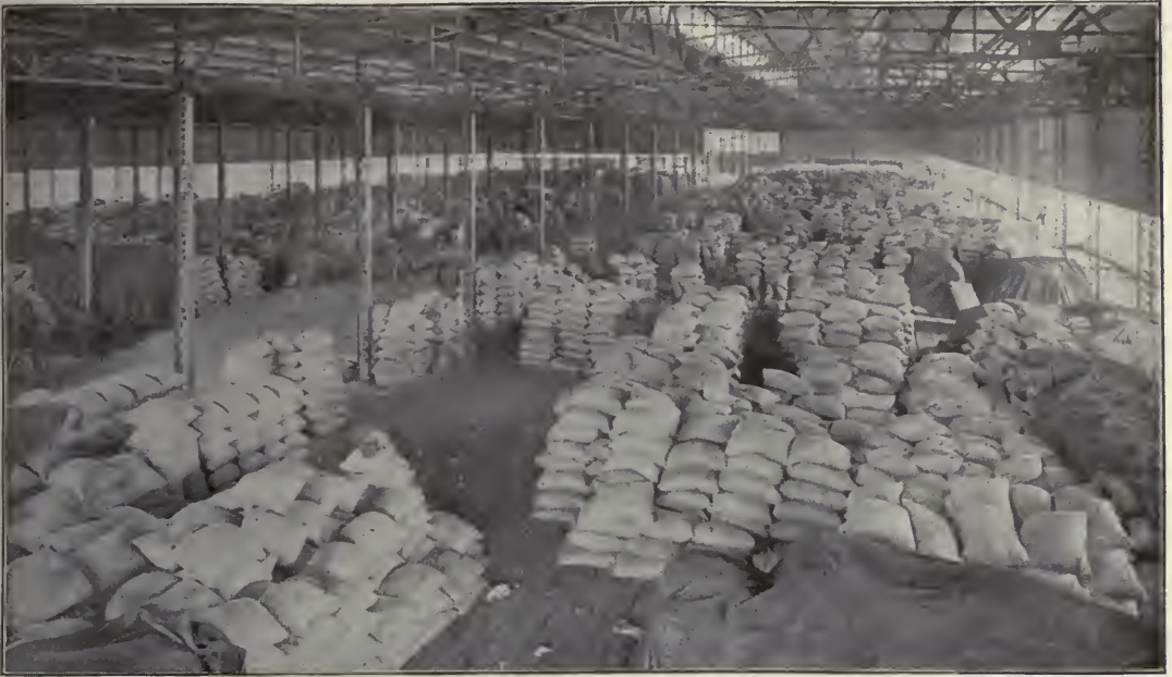
SHOWING HOW COFFEE IS STORED UNDER STEEL-COVERED SHEDS AT NEW ORLEANS
