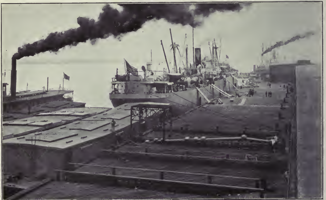
IN FOREGROUND — LOADING COFFEE BY MEANS OF AN AUTOMATIC TRAVELING-BELT CONVEYOR, ON GOVERNMENT BARGES FOR ST. LOUIS
