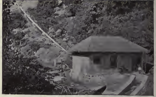
Hydro-electric power plant on Finca Ona.
