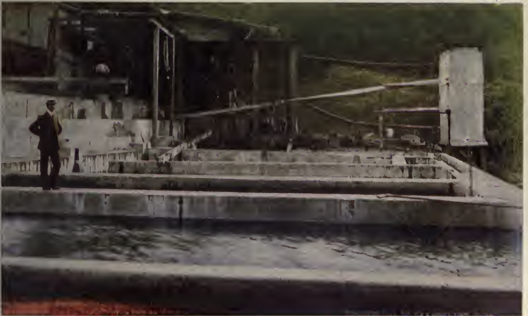
PULPING HOUSE AND FERMENTATION TANKS, COSTA RICA
