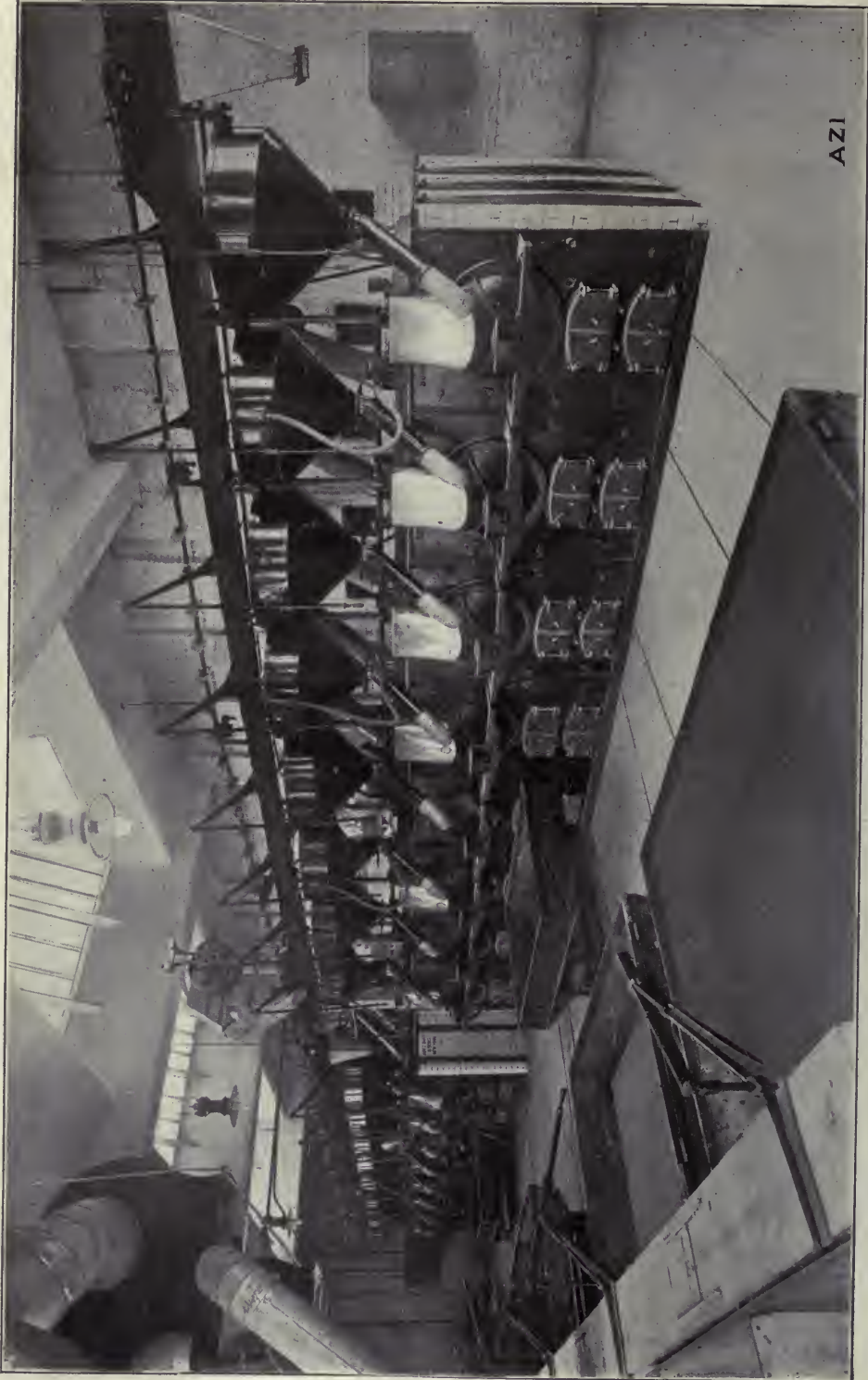
A SIXTEEN-CYLINDER COAL ROASTING PLANT IN A NEW YORK FACTORY This is a view of the roasting room of B. Fischer & Co. and shows a battery of Burns coal roasters
