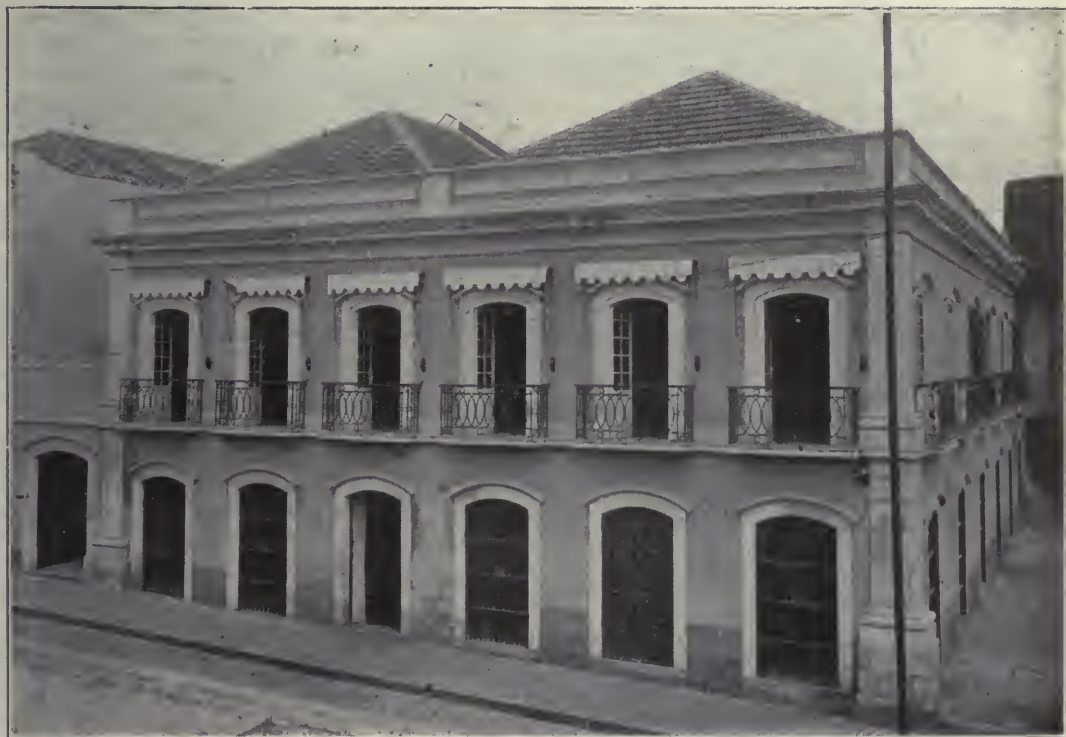
HAND & RAND BUILDING: FIRST FLOOR, STORAGE; SECOND FLOOR, OFFICES NEW YORK COFFEE IMPORTERS' MODEL ESTABLISHMENT AT SANTOS
