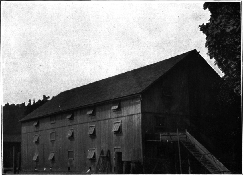
FIG. 1.—A THREE-STORY LAYING AND FATTENING HOUSE.
