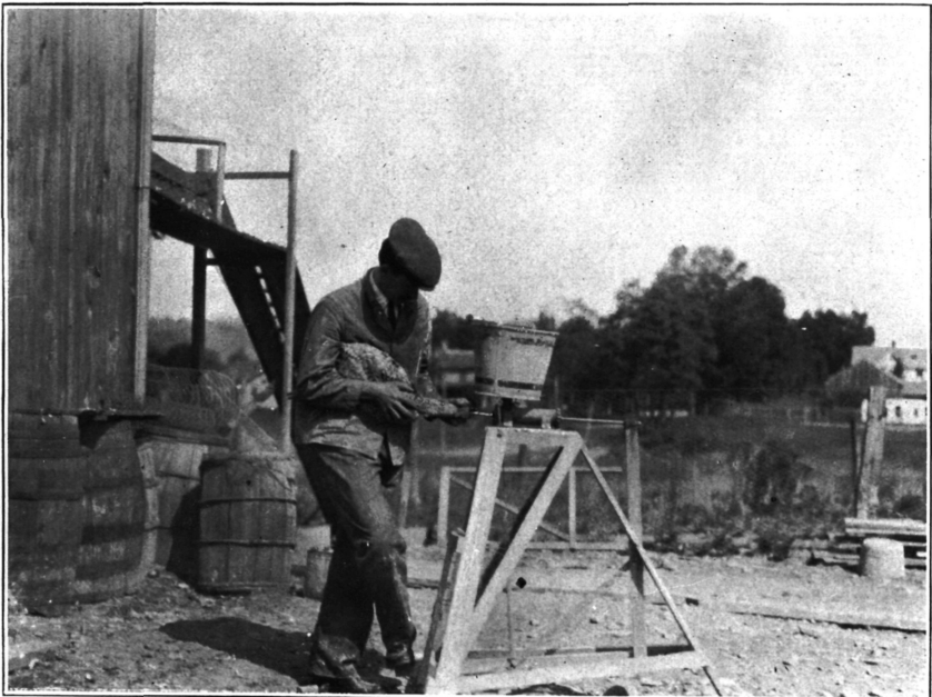
FIG. 2.—CRAMMING MACHINE IN OPERATION.
