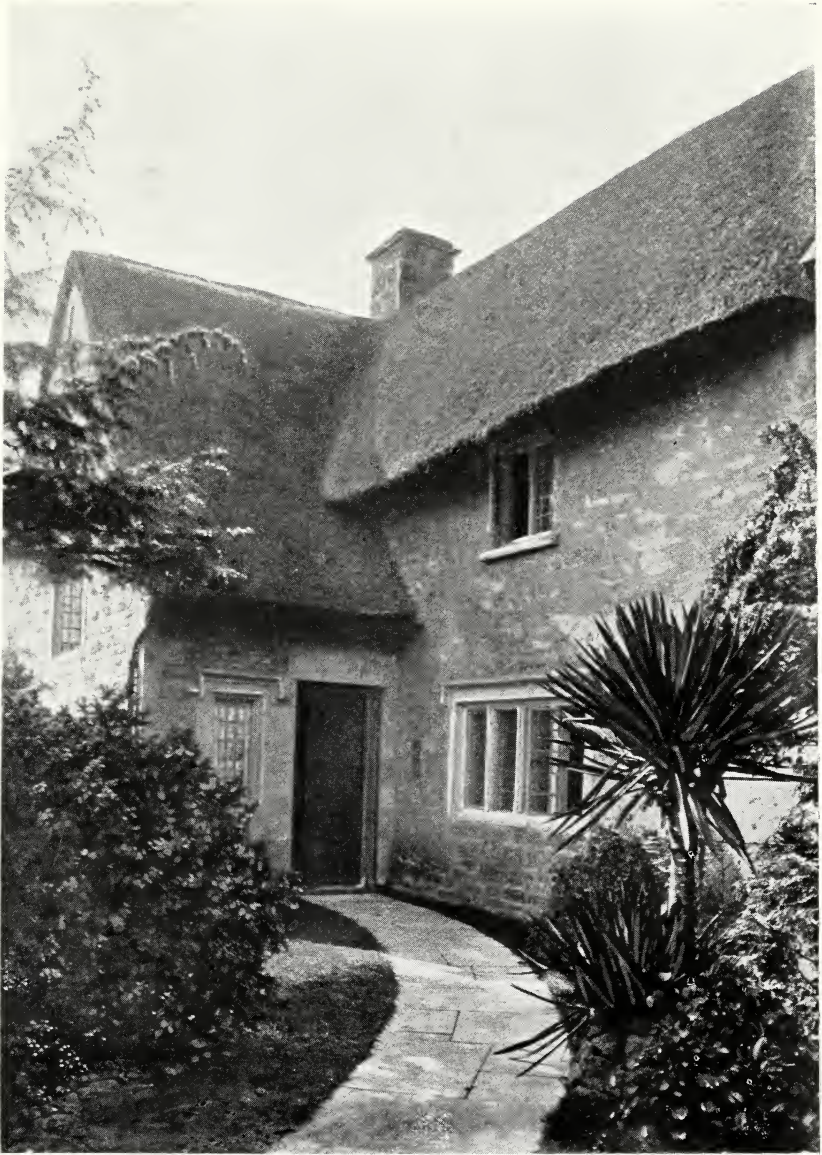
Appendix No. 15. Thatched Cottage at Westington.
