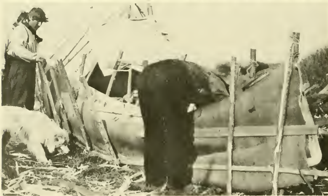
Assembling bark over on building site.
