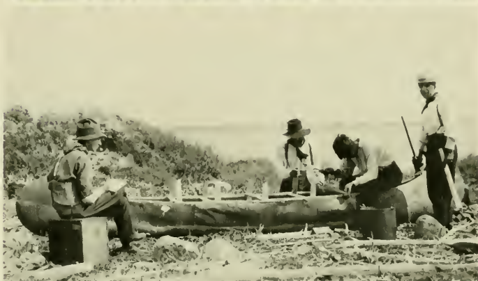
Setting ribs inside bark cover with a mallet.
