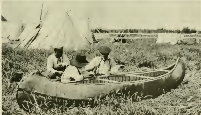
Fitting gunwale caps on new canoe.
