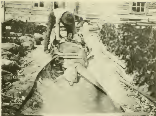
Weighting gunwales on bark cover on building bed.
